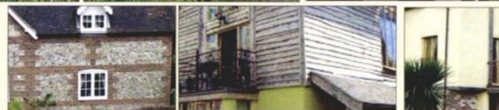
Clockwise from top: red brick, red clay roof tiles; black clay roof tile; timber cladding, timber with render and flint
