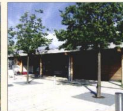
Small starter units Green Park, Reading
