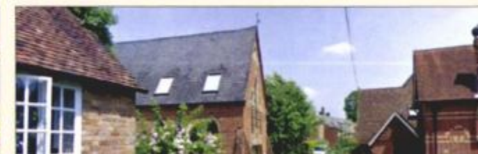
Gable end roofs in Cherton along the lanes
