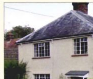
Hipped roof in Cherton
