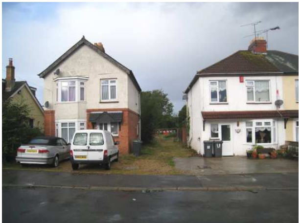
The application site viewed from Forest Avenue (east)
