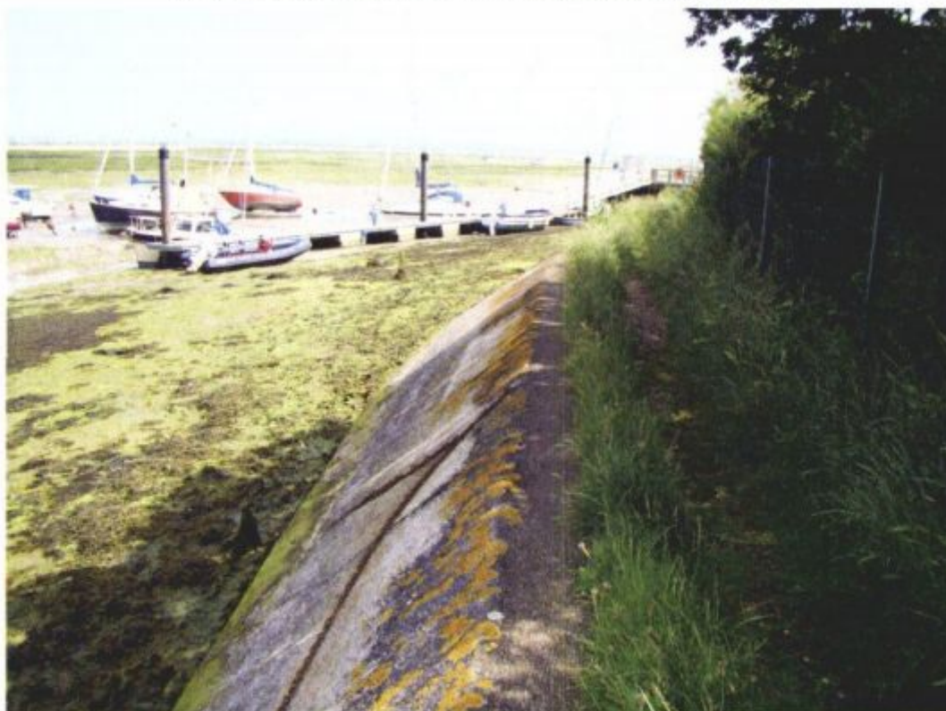
Photo 2: Access limited to SPA by steep banks along public footpath
