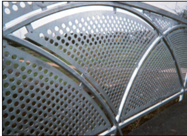
Figure 0-1 Typical Example of Open Screening formed from perforated steel panels.
