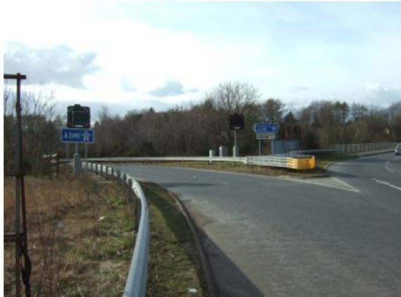
Figure 7. Crash Cushion at A3(M) Junction 3 Southbound On-slip
