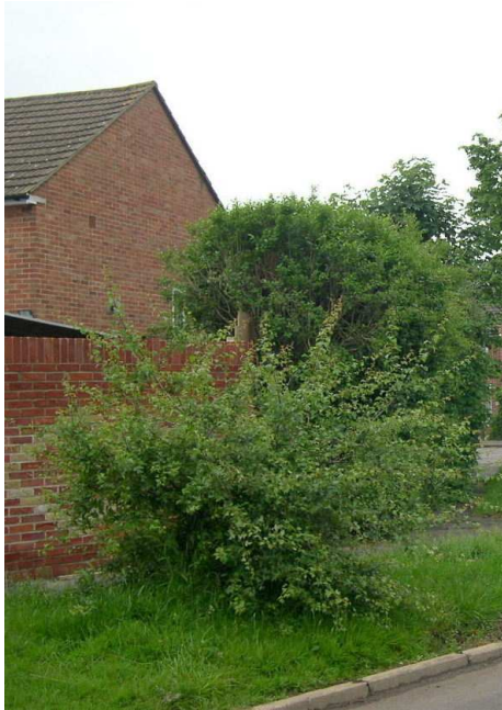
Photograph 3 - Taken from Hordle Road showing the existing boundary wall which is 2.2m high and is required to be extended along the new boundary line.
