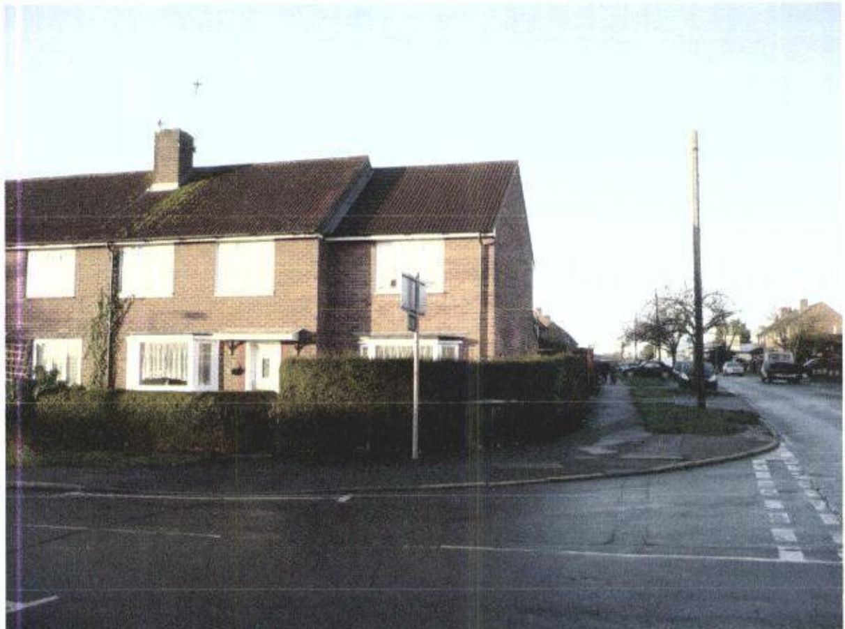
New dwelling at 2 James Road, Havant
