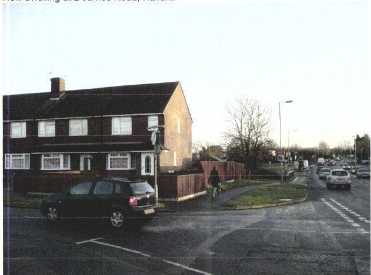
New dwelling at 25 James Road, Havant
