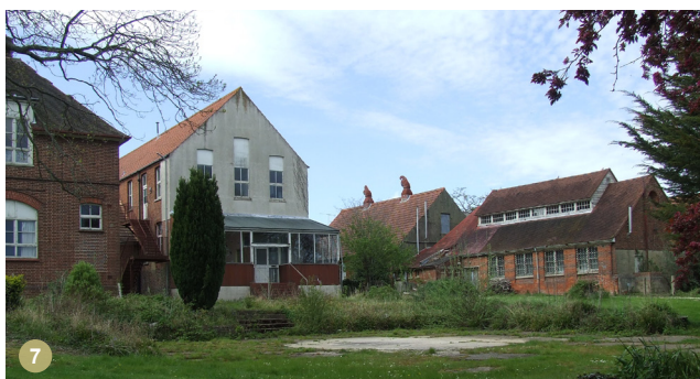
7 Extensions to the northern side elevation of the Convent (rear)
