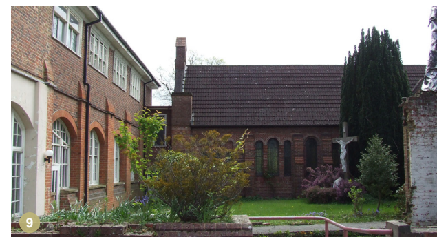
9 Former Convent and Chapel and cross
