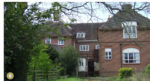
6 Extensions to the rear of St Michael's Convent
