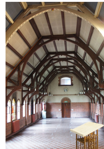
North nave with open timber hammer-beam roof
