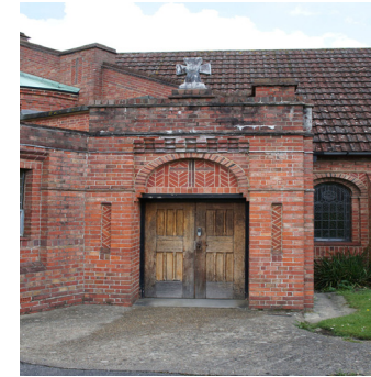
Herringbone patterns set into the exterior brickwork and English bond fletton brickwork
