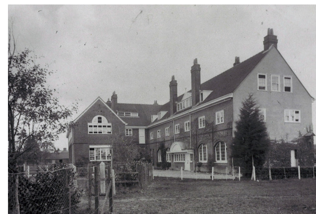
View of the northern end of the convent building including rendered gable
