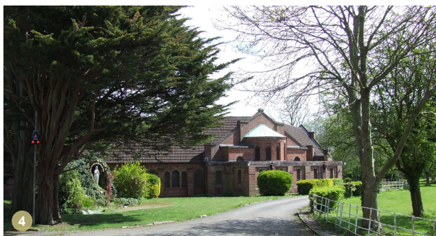
Mature trees around buildings
