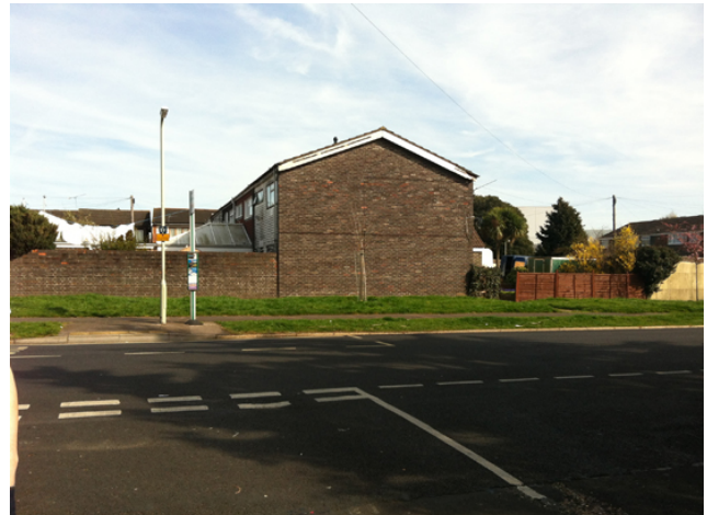
Figure 10: The gable ends of the terraces to Kyto walk form a very prominent feature of the street scene opposite No. 9 St Albans Road
