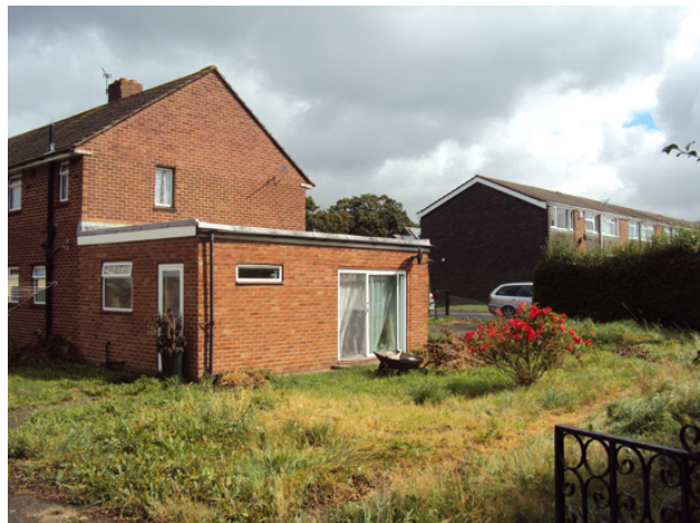
Figure 4: Views to the east of the differing style of later terraces (the single storey side extension that is proposed for demolition is shown here within the proposed site)
