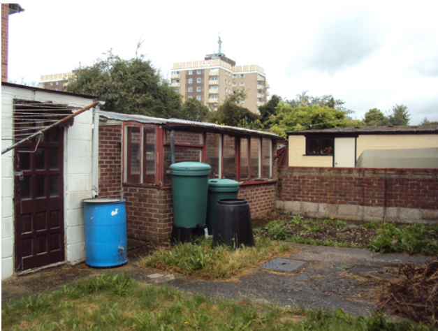
Figure 3: Views to the north of No. 9 are dominated by tower blocks (the white garage proposed for demolition is shown to the left)
