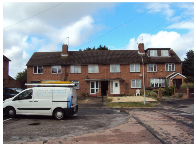
Figure 12: A terrace in Dunhurst Close with an incongruous corner unit – large extension to the roof and an untypically large porch
