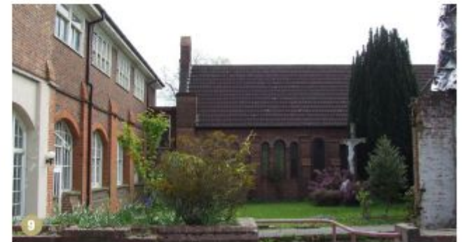
Former Convent and Chapel and cross
