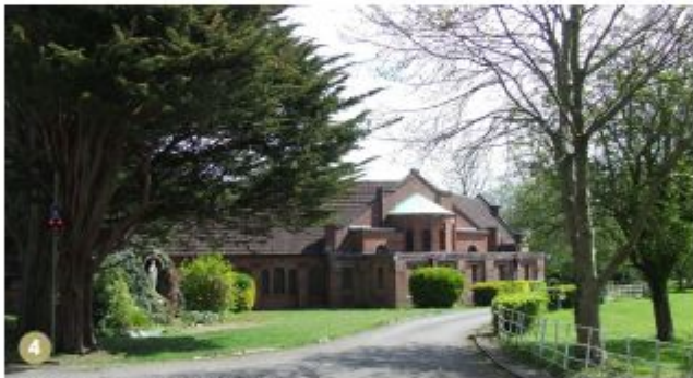
4 Mature trees around buildings
