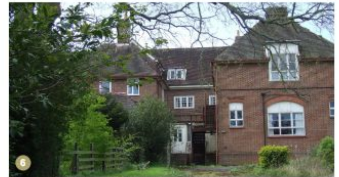
Extensions to the rear of St Michael's Convent
