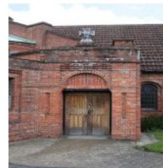
Herringbone patterns set into the exterior brickwork and English bond fleton brickwork
