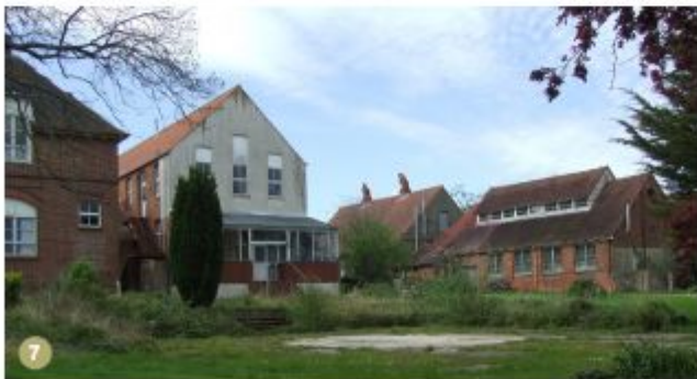
Extensions to the northern side elevation of the Convent (rear)
