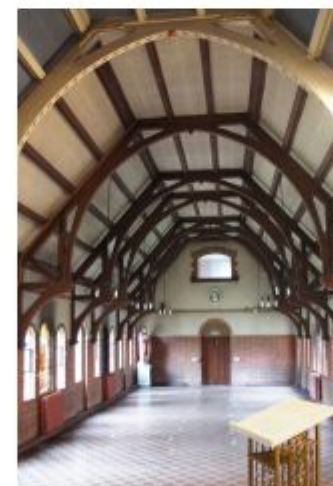
North nave with open timber hammer-beam roof
