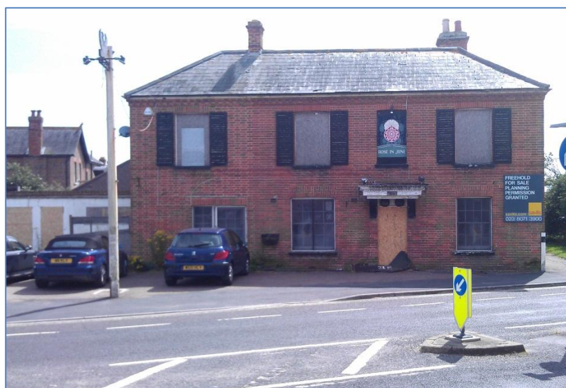
Photograph 1 Existing Development: The Rose in June
