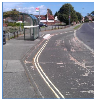
Photograph 6 Vehicle Crossover for Servicing
