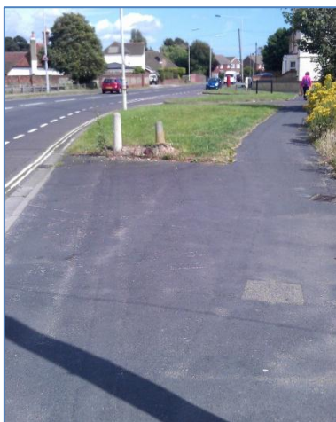
Photograph 10 Footway fronting the site
