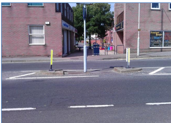
Photograph 5 Selsmore Road Traffic Splitter Island
