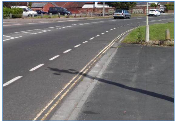
Photograph 4 Carriageway margin on Selsmore Rd.
