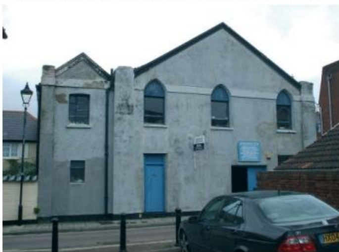
Figure 5: Front elevation of existing building
