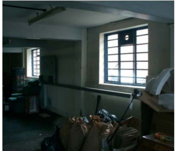
Figure 3: Inside showing concrete floors and beams and metal windows
