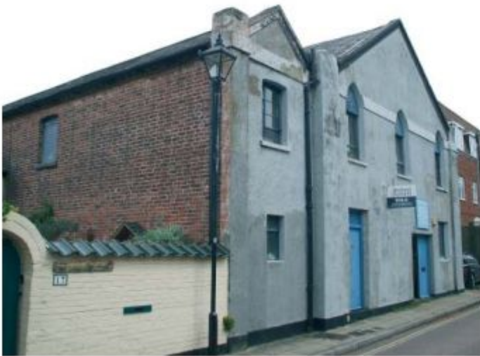
Figure 2: Frontage to Nile Street showing altered fenestration
