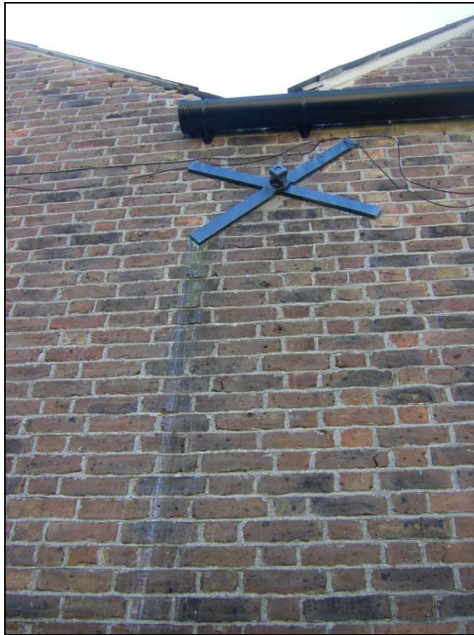
Photo 3: North elevation at junction of the two pitched roofs. The pattrress plate attached to the tie bar is clearly visible.
