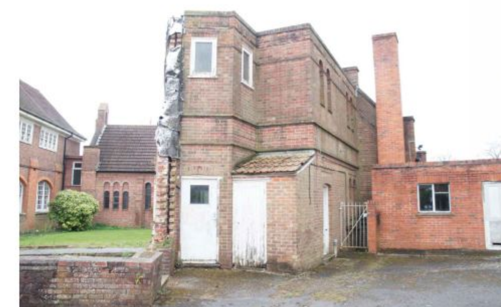
VIEW OF NORTH EAST GABLE WALL OF THE CHURCH, THE PARTIALLY DEMOLISHED TWO STOREY LINK BUILDING AND THE SINGLE STOREY BOILER HOUSE AND CHIMNEY FROM THE NORTH
