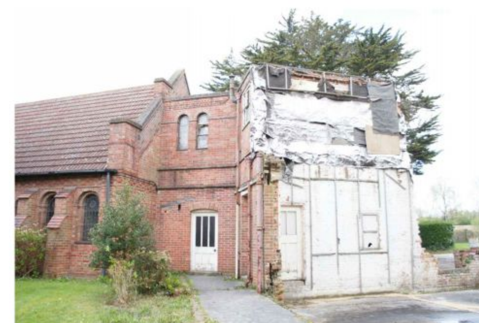
VIEW OF NORTH EAST GABLE WALL OF THE CHURCH AND PARTIALLY DEMOLISHED TWO STOREY LINK BUILDING FROM THE EAST
