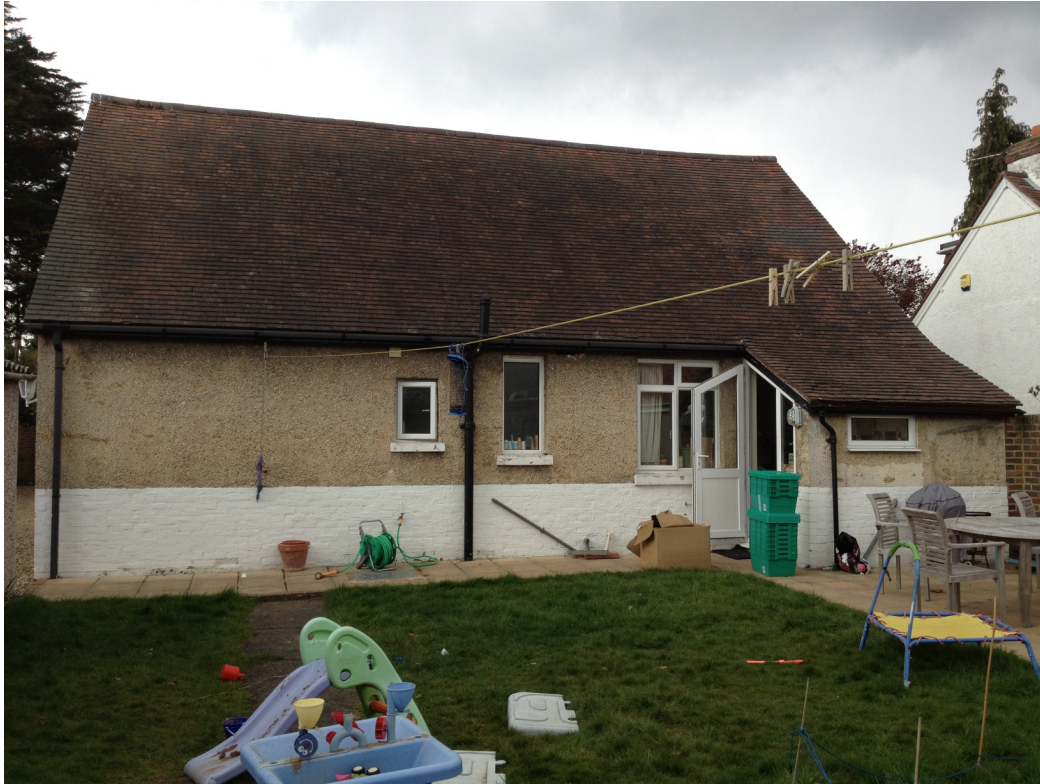
Fig 2: Existing Rear Elevation
