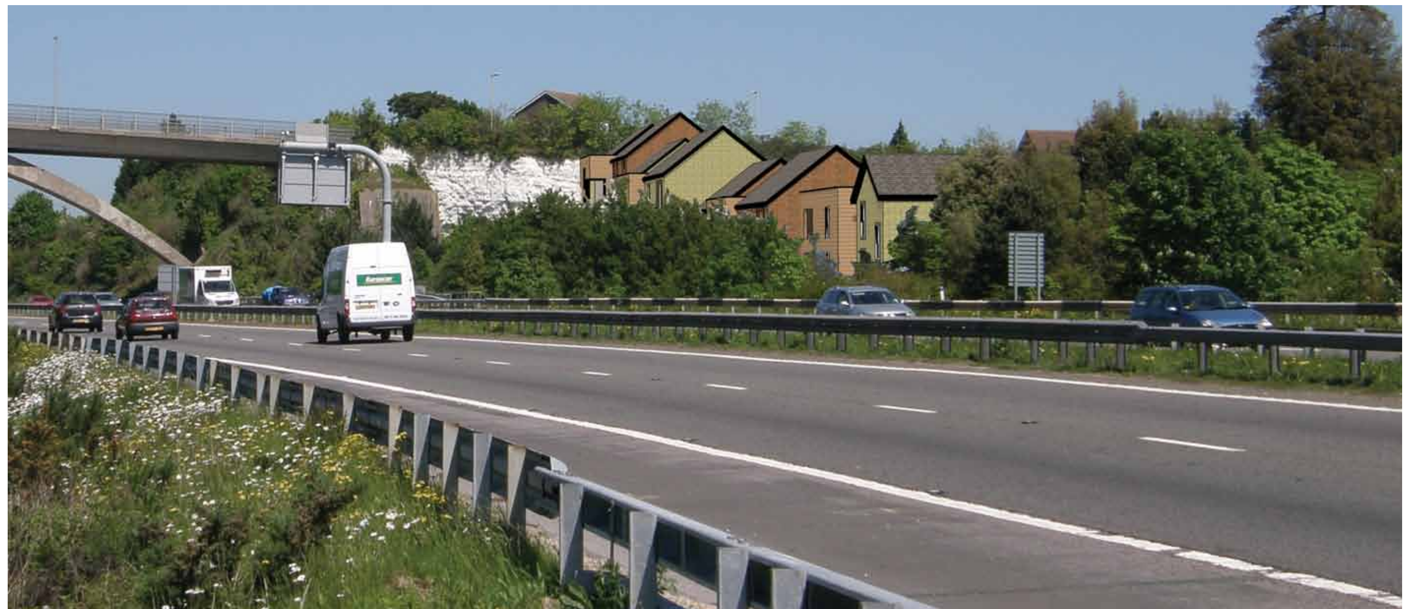
View of 'barrier block' from the A3(M)
