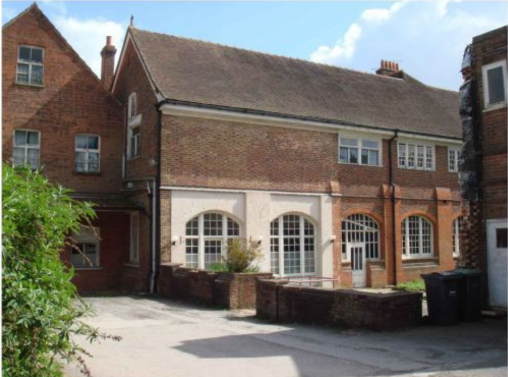
CURRENT VIEW OF AREA SHOWN IN PHOTO ABOVE, LOOKING FROM THE NORTH WEST SHOWING THE PARTIALLY DEMOLISHED LINK BUILDING IN RIGHTHAND FOREGROUND
