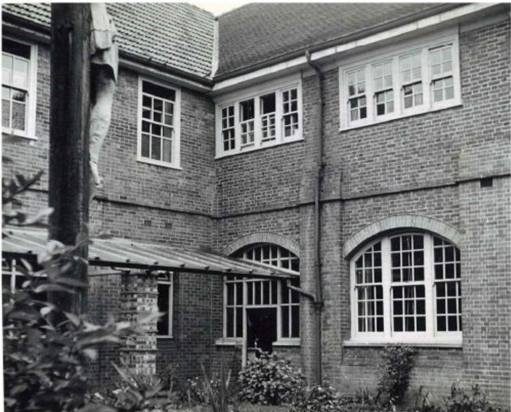
VIEW OF ST MICHAEL'S CONVENT SHOWING THE TWO STOREY LINK BUILDING THAT CONNECTED TO THE CHURCH OF THE SACRED HEART (NOW PARTIALLY DEMOLISHED)
