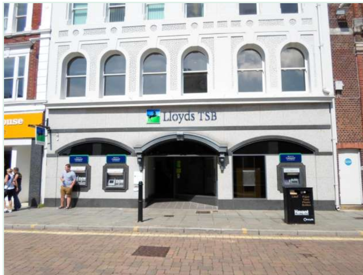
EXISTING SIGNAGE OVERVIEW
