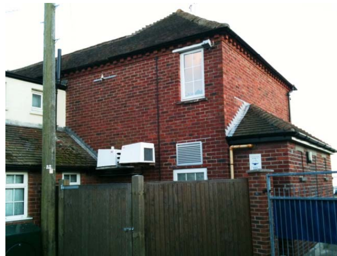
Front of clubhouse – detail of east extensions
