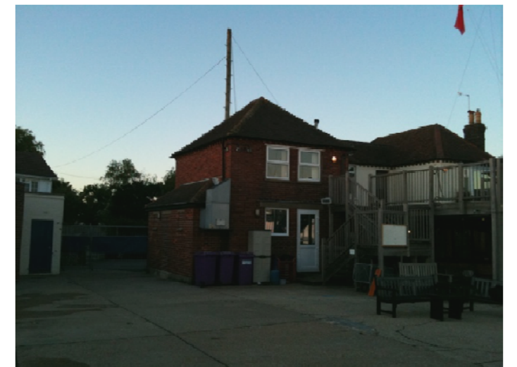
View from jetty – detail of east extensions
