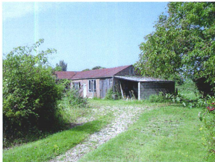
The existing stable block on land to the North of the retreat
