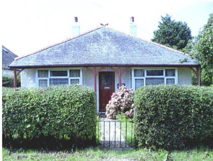
The Existing Building – ‘The Retreat’
