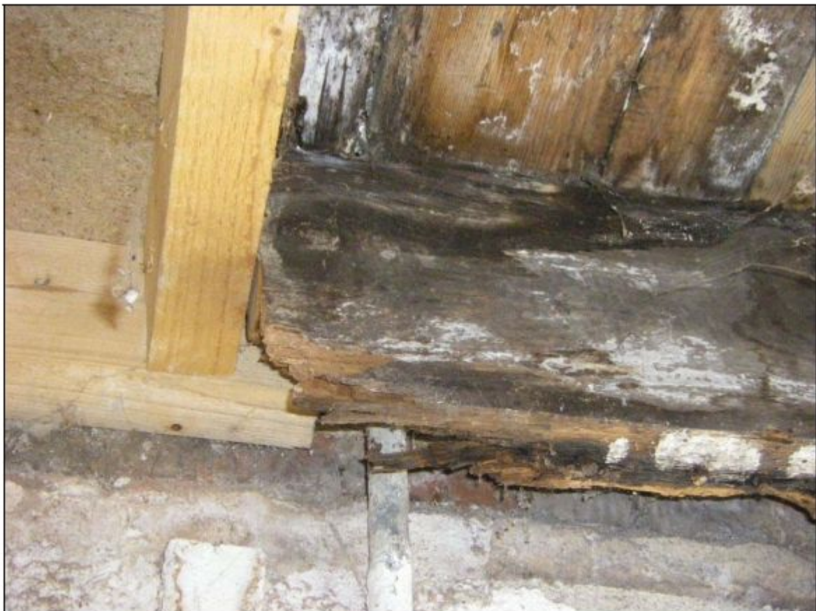
Photo 6: Repair to first floor joist, decayed timber still visible.
