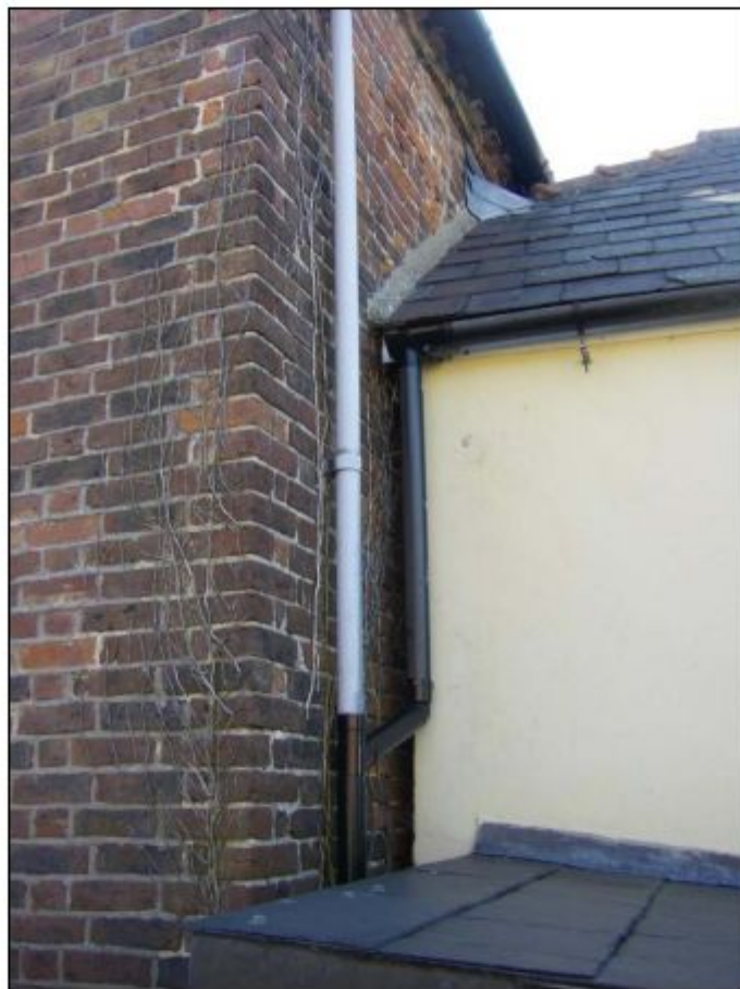
Photo 4: Abutment of adjoining property and the west elevation.
