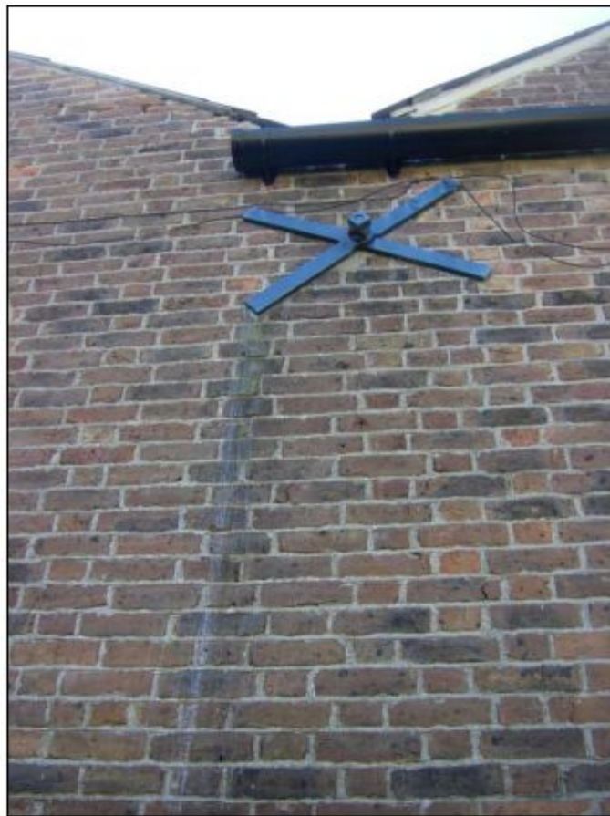
Photo 3: North elevation at junction of the two pitched roofs. The pattern plate attached to the tie bar is clearly visible.
