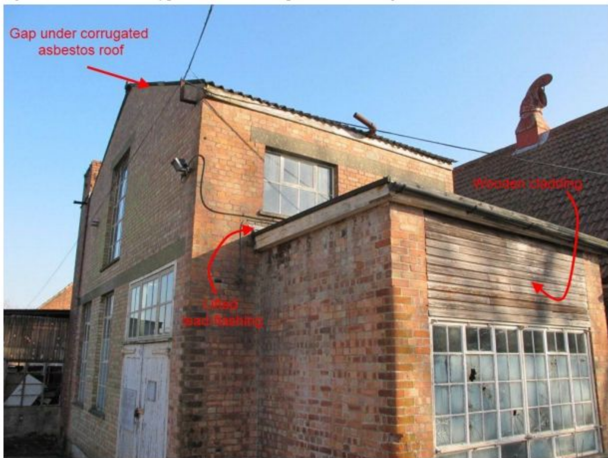
Figure C.7.1.1. Location of potential bat access points on Building A.
