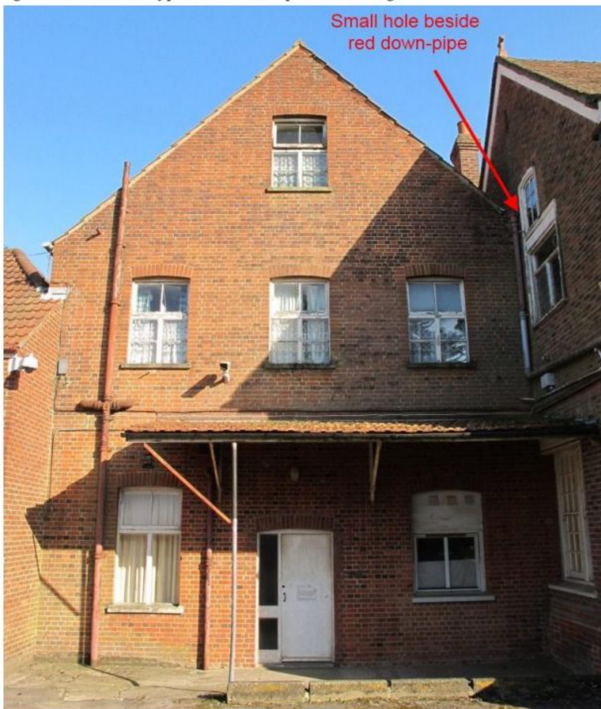
Figure C.7.1.9. Location of potential bat access points on Building E.
