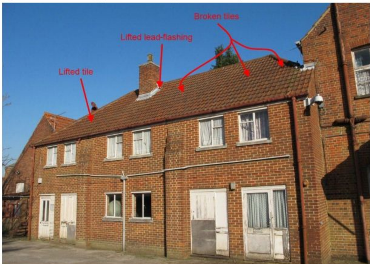
Figure C.7.1.8. Location of potential bat access points on Building C.
