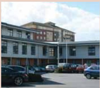
Internal parking court at Basepoint
