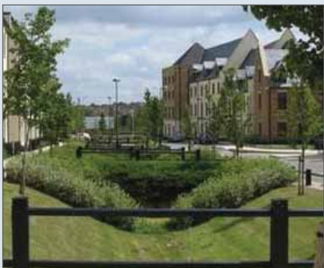
Sustainable urban drainage system, Upton
