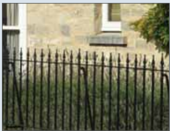
Metal railings to front property boundaries
