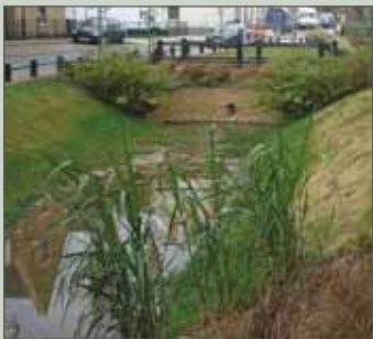
SuDS and river restoration
