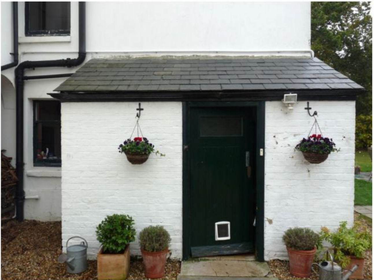
Queensberry Lodge, 15 Hollow Lane, Boot Lobby
