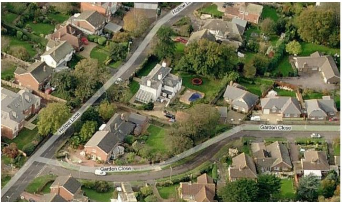
Queensberry Lodge viewed from North East
