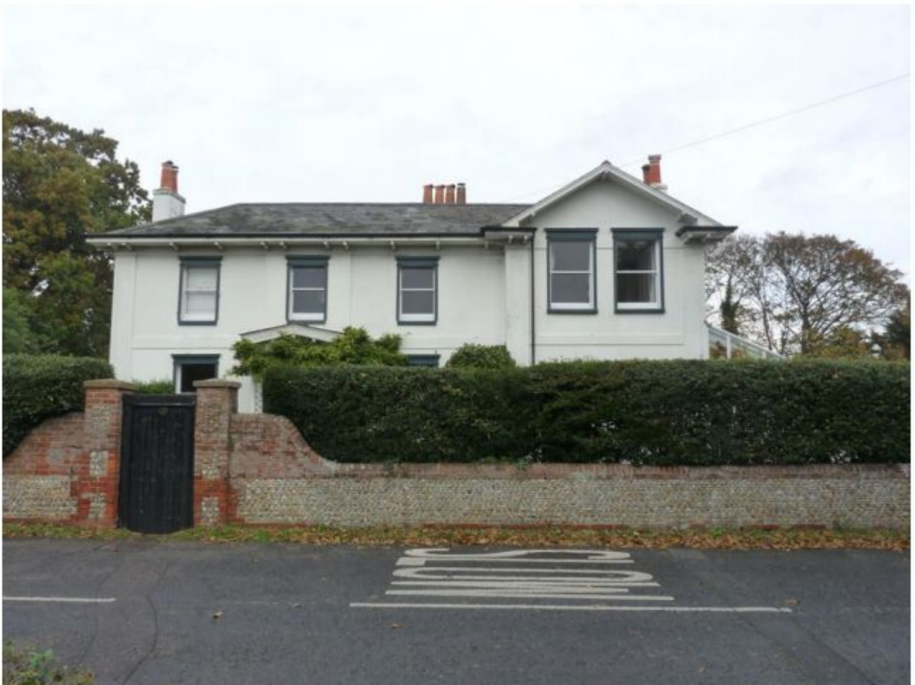
Queensberry Lodge, 15 Hollow Lane, facing South West
