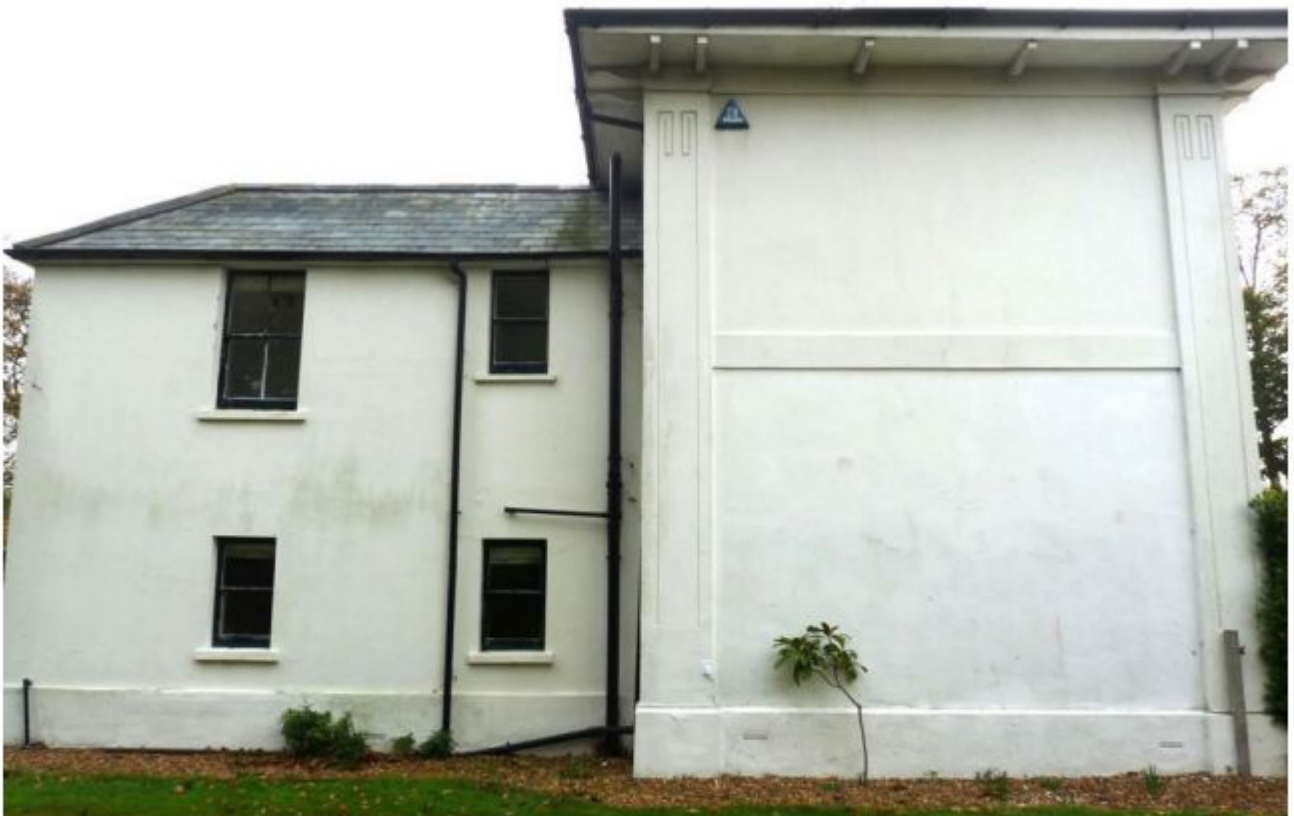
Queensberry Lodge, 15 Hollow Lane, facing North West
