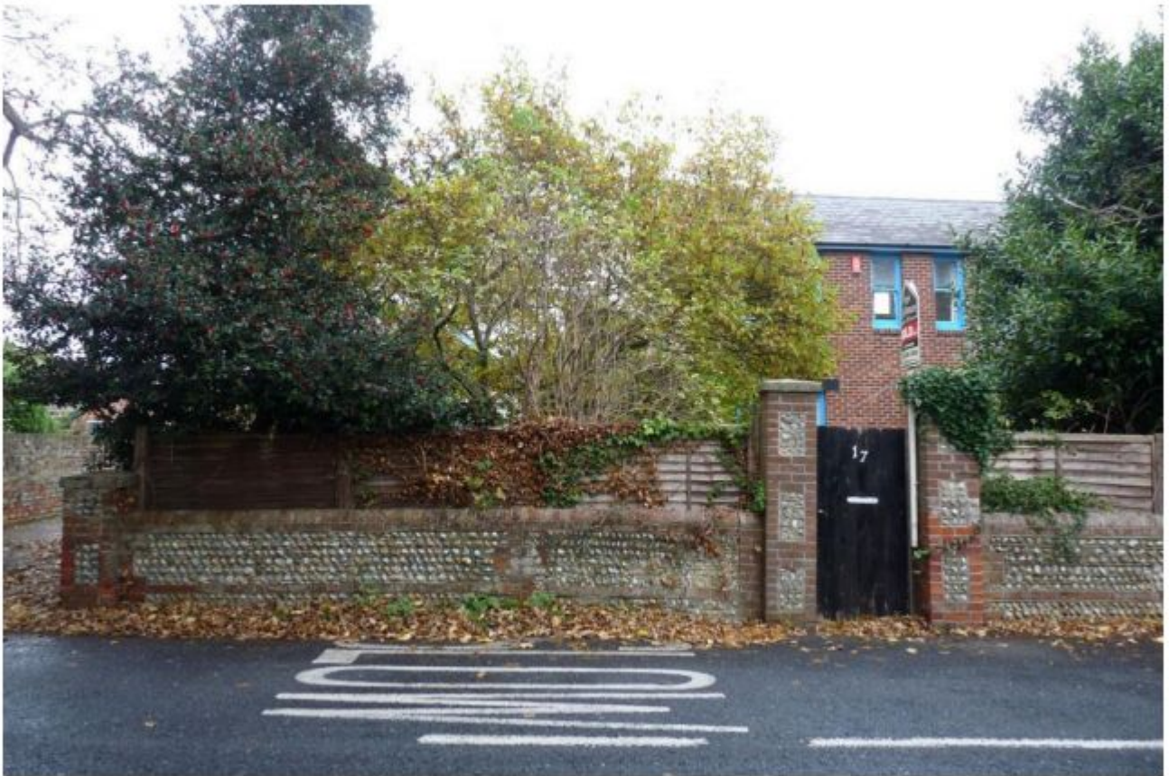
17 Hollow Lane (currently being extended)
