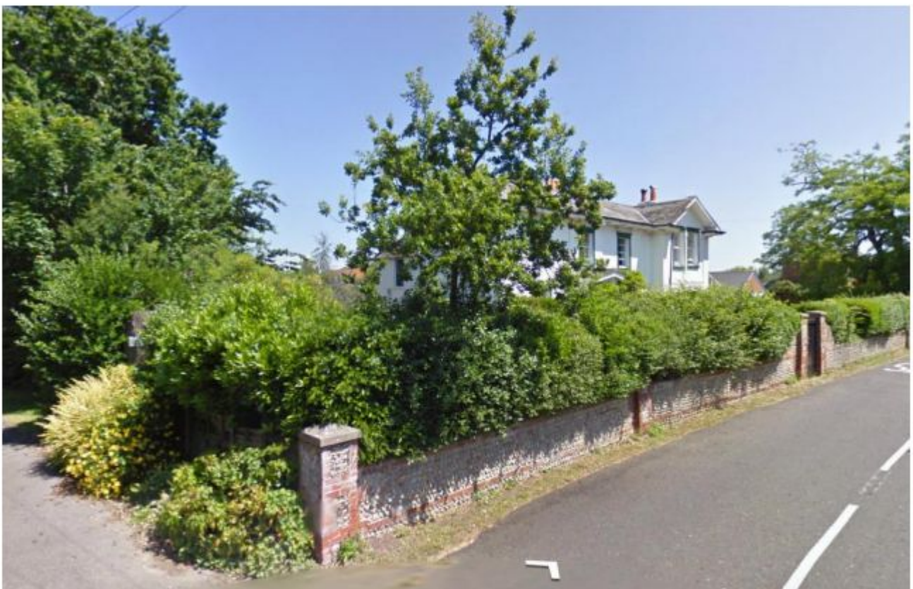
Street view of Queensberry Lodge, on Hollow Lane
