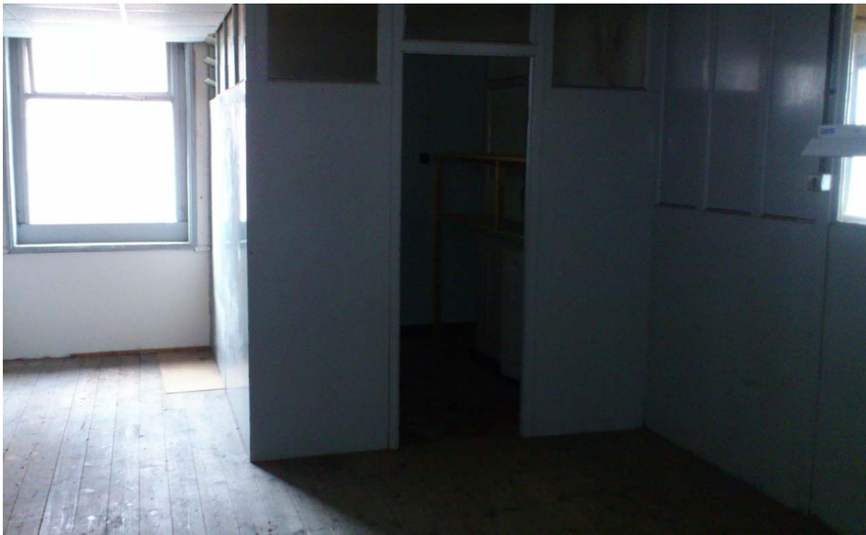
Photograph No. 10 - Office spaces on the first floor, with 'Nil' Bat Roost Potential.
