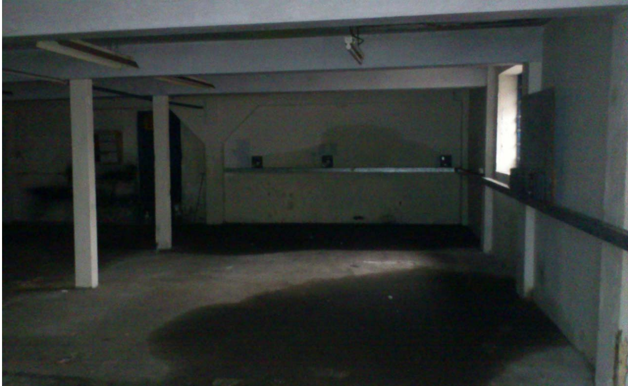
Photograph No. 1 - Ground floor - Photograph taken from the main access door looking northward. The room is relatively light, with no access points for bats, minimal suitable crevices / cavities for bats, and 'Nil' Bat Roost Potential.
