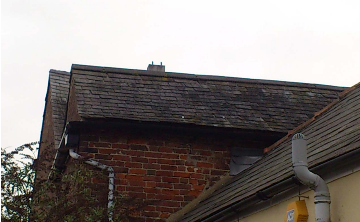
Photograph No. 19 - Western elevation of the existing building. Tiles are tight-fitting slate with minimal potential access points exist under the eaves. In the local context this equates to 'Negligible' Bat Roost Potential.
