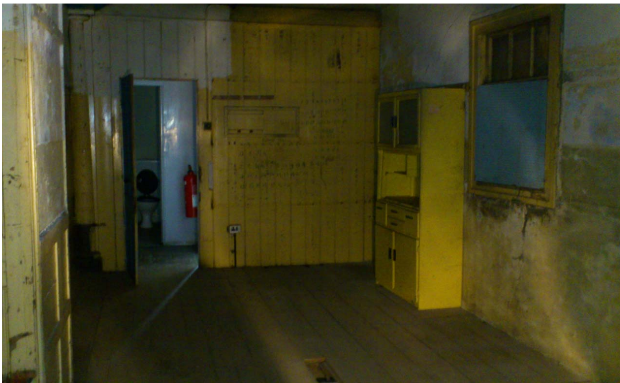
Photograph No. 6 - Kitchen / dining area on the first floor, with no bat access and no viable bat roost space, and 'Nil' Bat Roost Potential.
