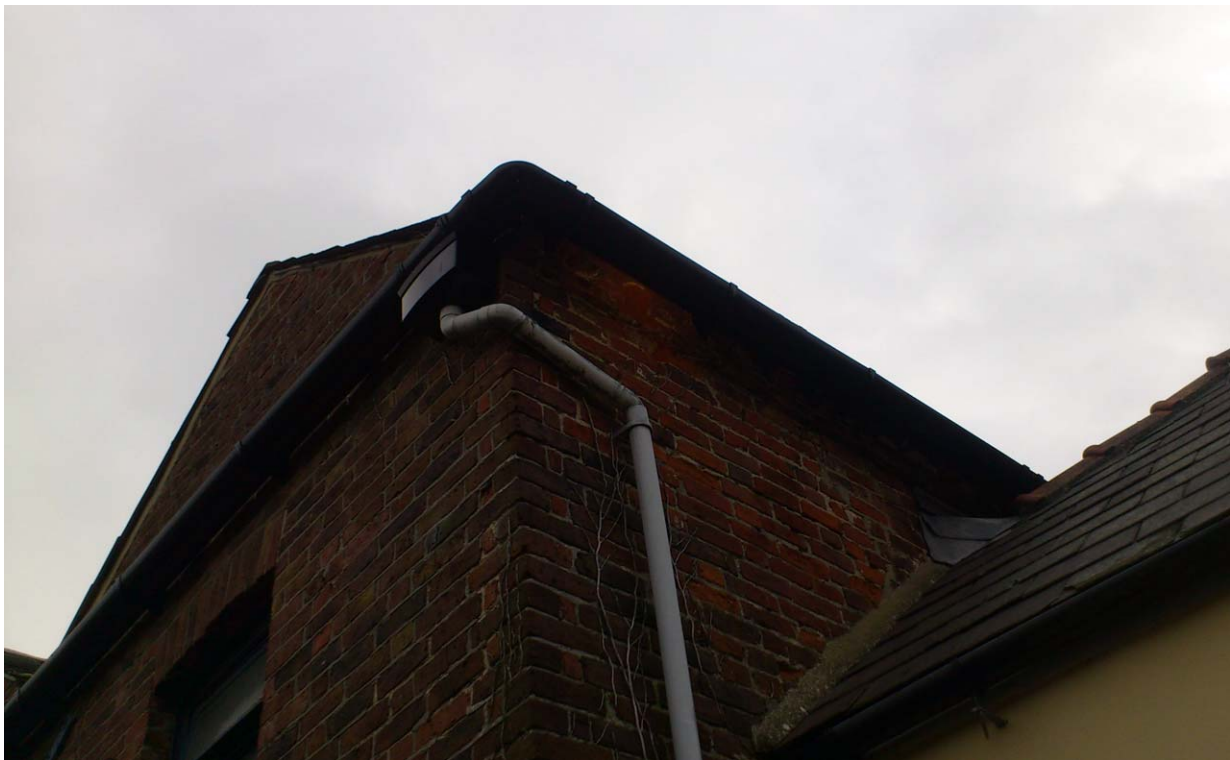
Photograph No. 20 - Minimal potential bat access points under the eaves on the western elevation.
