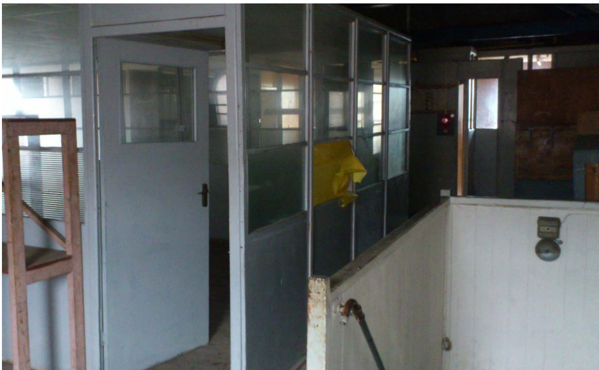
Photograph No. 8 - Office spaces on the first floor, with 'Nil' Bat Roost Potential.
