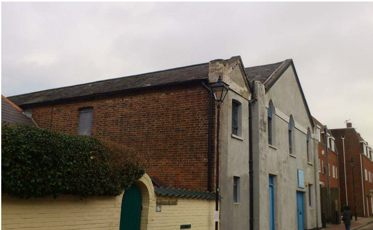
Photograph No. 22 - Tight-fitting slate tiles over all visible areas of the roof, with minimal bats access points, and 'Negligible' Bat Roost Potential.
