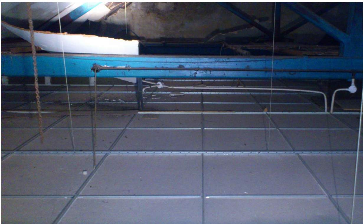
Photograph No. 12 - Roof space above the offices on the first floor. This area is conspicuously clean and free of any evidence of bat occupation. There is good access to the main loft void and is unlikely to have been cleaned.
