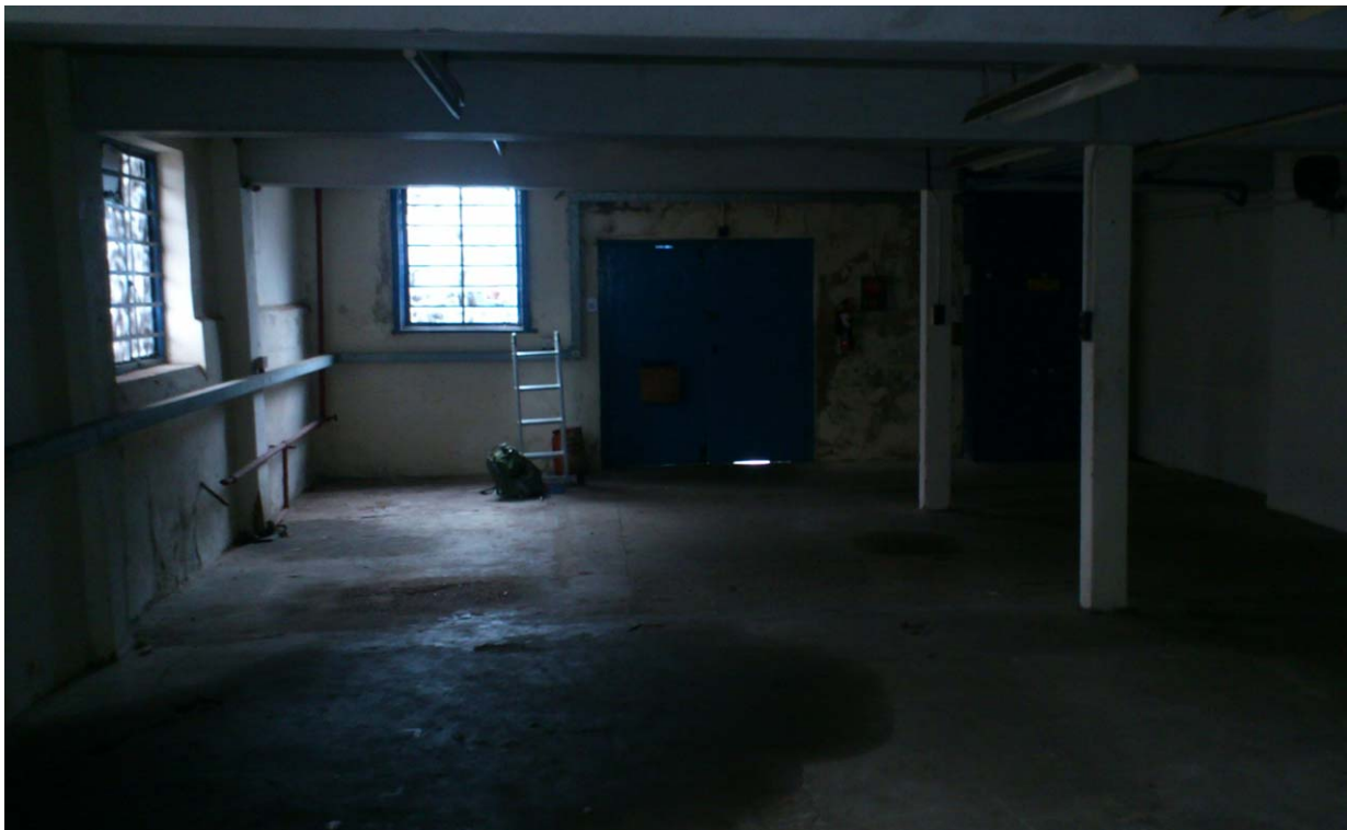
Photograph No. 2 - Ground floor - Photograph taken from the northern wall looking eastward. the room is relatively light, with no access points for bats, minimal suitable crevices / cavities for bats, and 'Nil' Bat Roost Potential.
