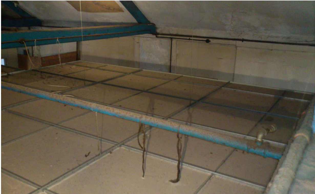
Photograph No. 13 - Southern area of roof space above offices on first floor. The area is clean and free of any evidence of bat occupation. There is good access to the main loft void and is unlikely to have been cleaned.
