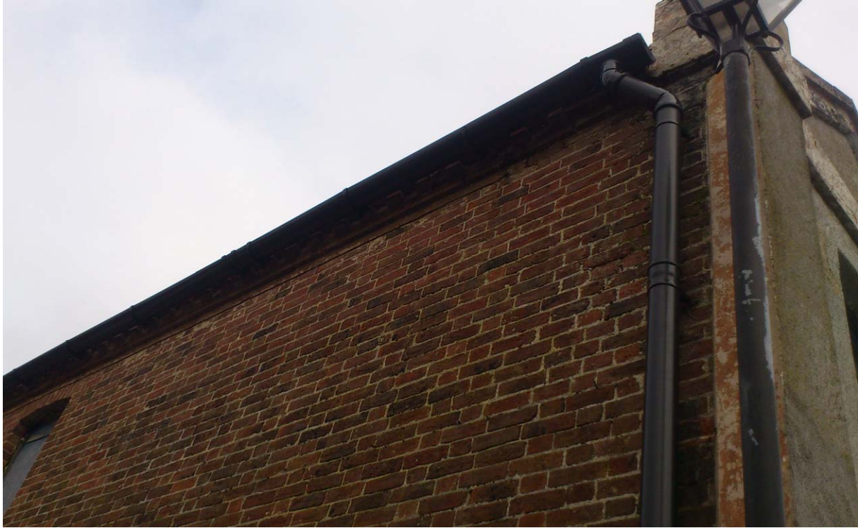
Photograph No. 21 - Minimal potential bat access points under the eaves on the western elevation.
