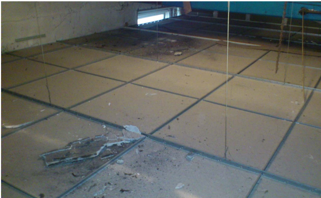
Photograph No. 14 - Northern area of roof space to offices on the first floor. This area is clean and free of any evidence of bat occupation. There is good access to the main loft void and is unlikely to have been cleaned.
