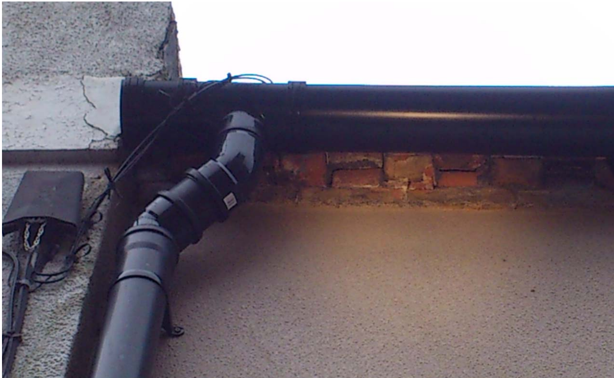
Photograph No. 16 - Potential bat access point around the roof eaves on the eastern elevation. In the local context equates to 'Negligible' Bat Roost Potential.
