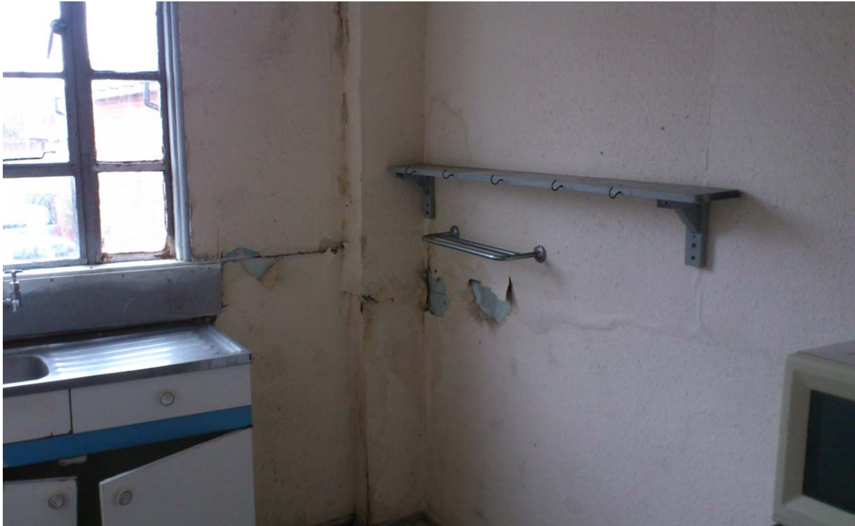
Photograph No. 7 - Utility room on the first floor, which is too light and not viable roosting space for bats, with 'Nil' Bat Roost Potential.
