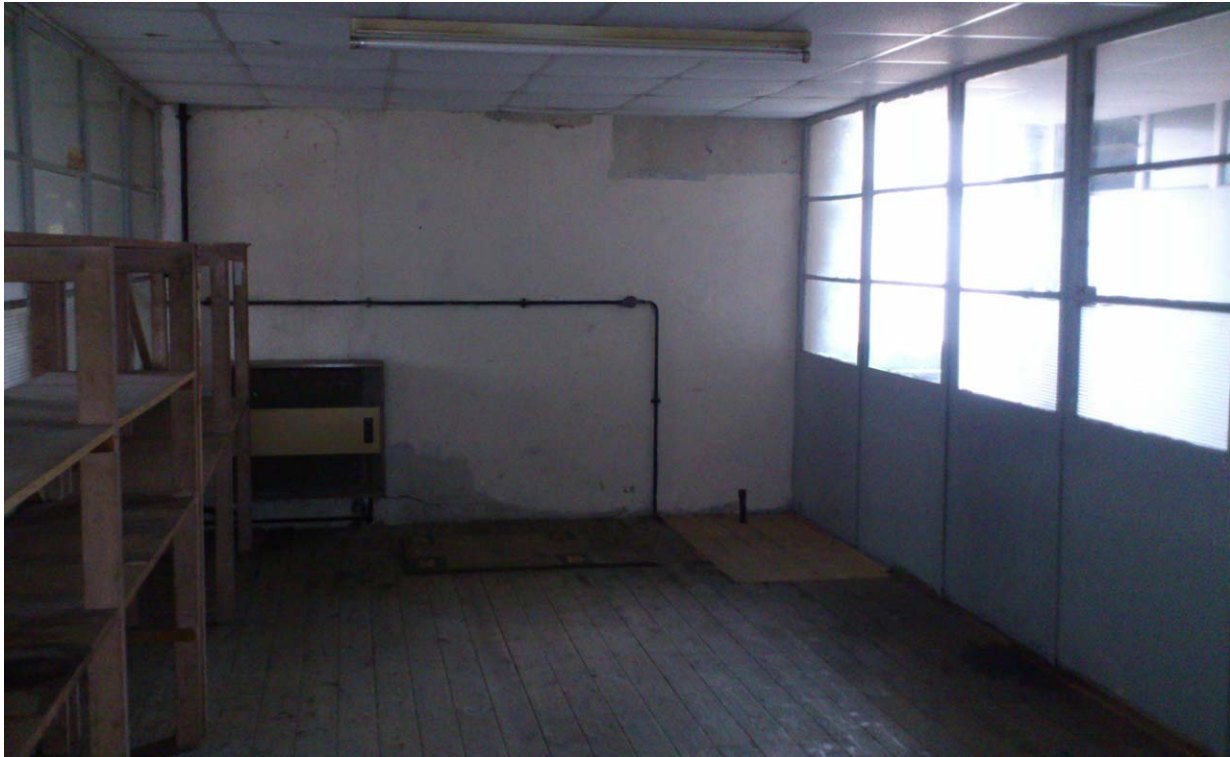
Photograph No. 9 - Office spaces on the first floor, with 'Nil' Bat Roost Potential.
