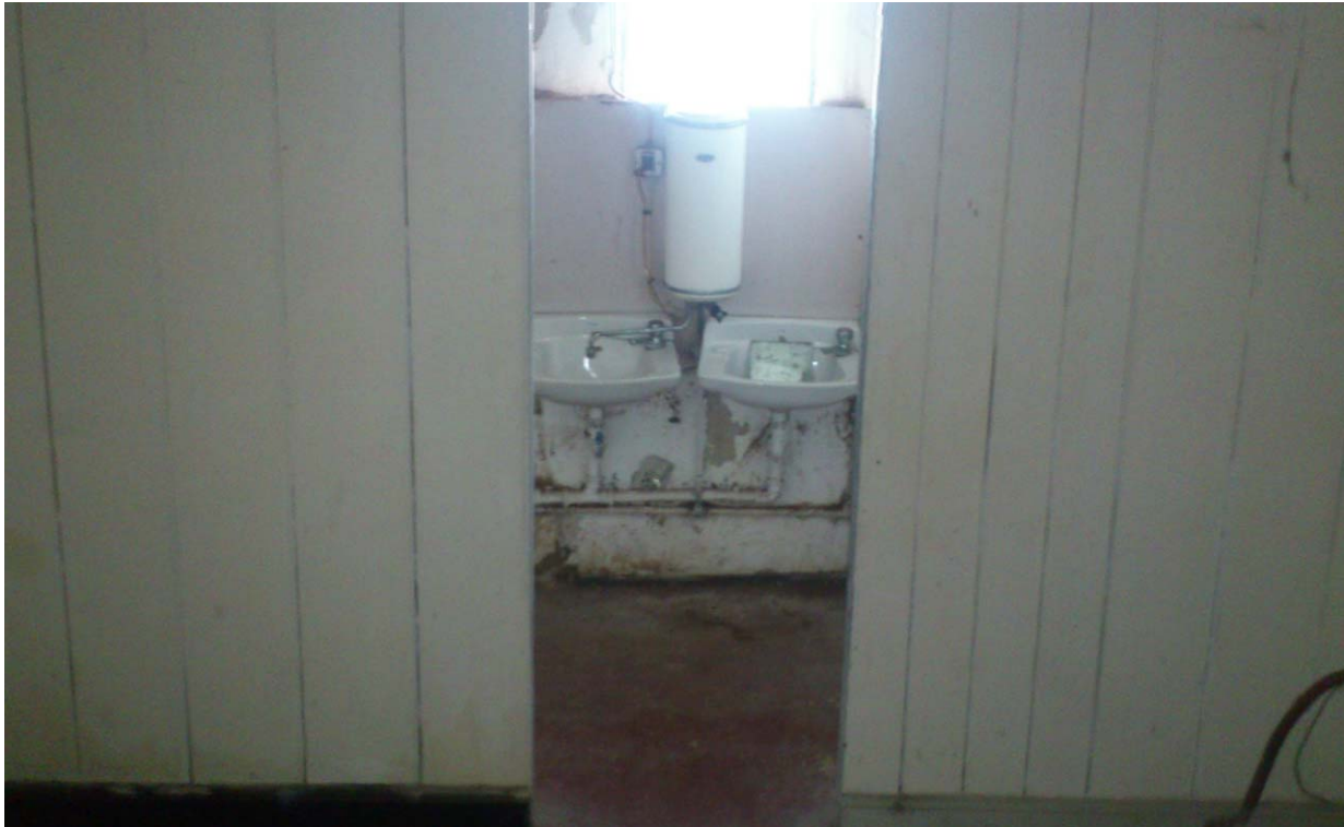
Photograph No. 5 - Toilet on the ground floor, which is too light for bats, with 'Nil' Bat Roost Potential.
