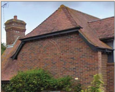
Half-Hipped roof in Cheriton
