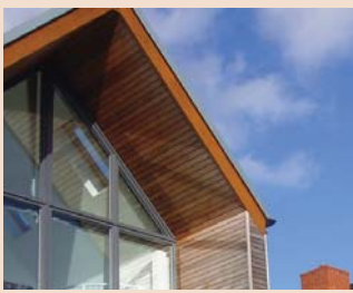
Eaves: Examples of deep eaves detail
