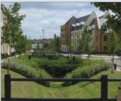
Sustainable urban drainage system, Upton
