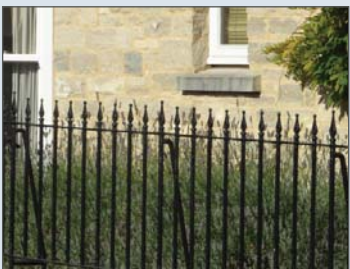
Metal railings to front property boundaries
