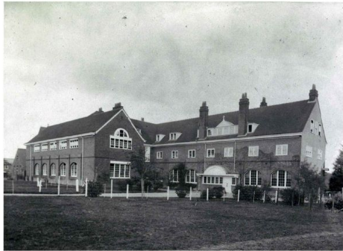
VIEW OF ST MICHAEL'S CONVENT FROM SOUTH WEST TAKEN PRIOR TO CONSTRUCTION OF THE CHURCH OF THE SACRED HEART SHOWING THE ORIGINAL CONVENT & RENDERED GABLE
