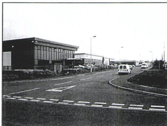
Industrial units in Southmoor Lane
