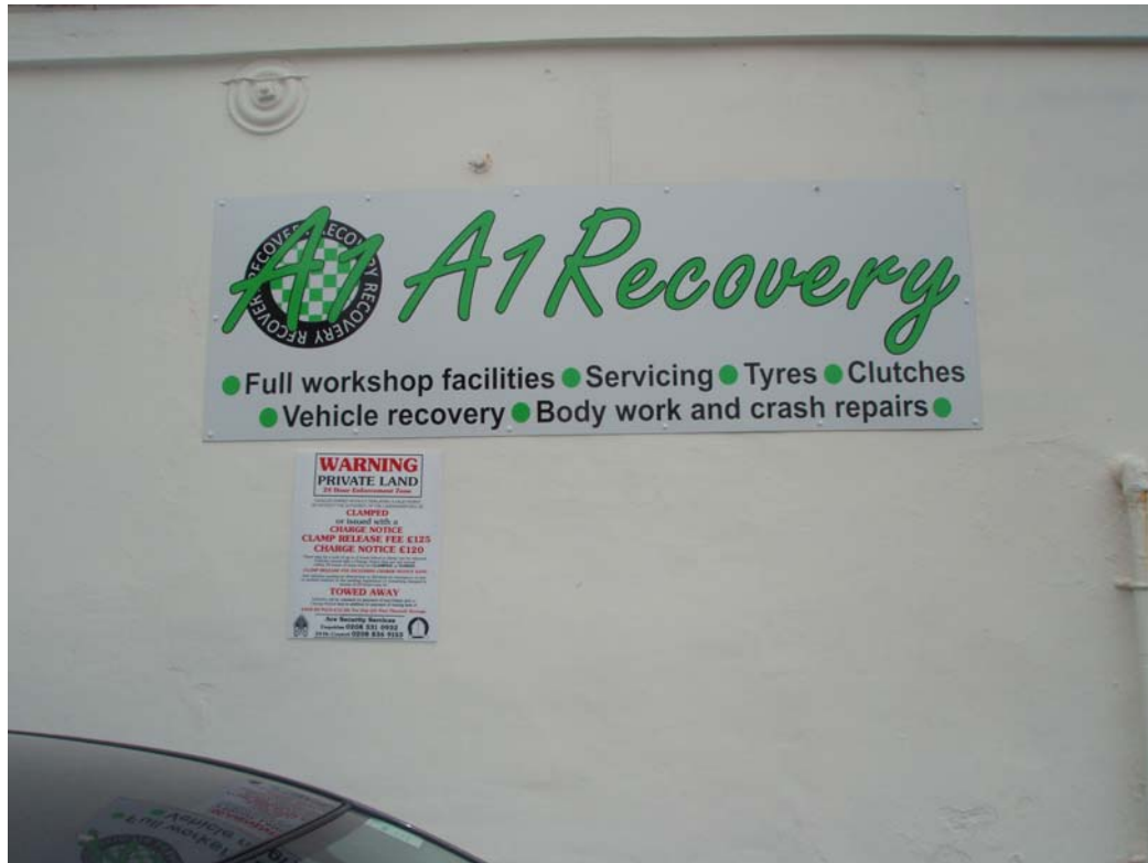
Photograph 8 –Signage on rear wall of Woodwork shop facing North.
