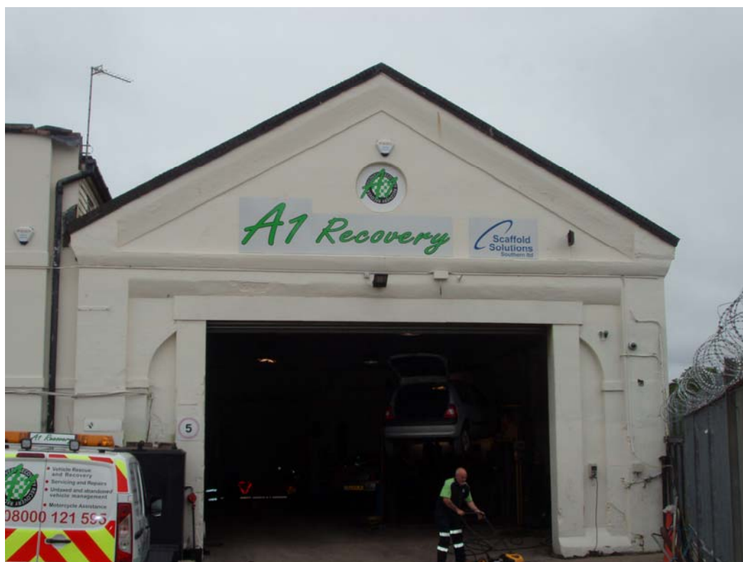
Photograph 11 – Signage on gable end wall of vehicle workshop facing North.
