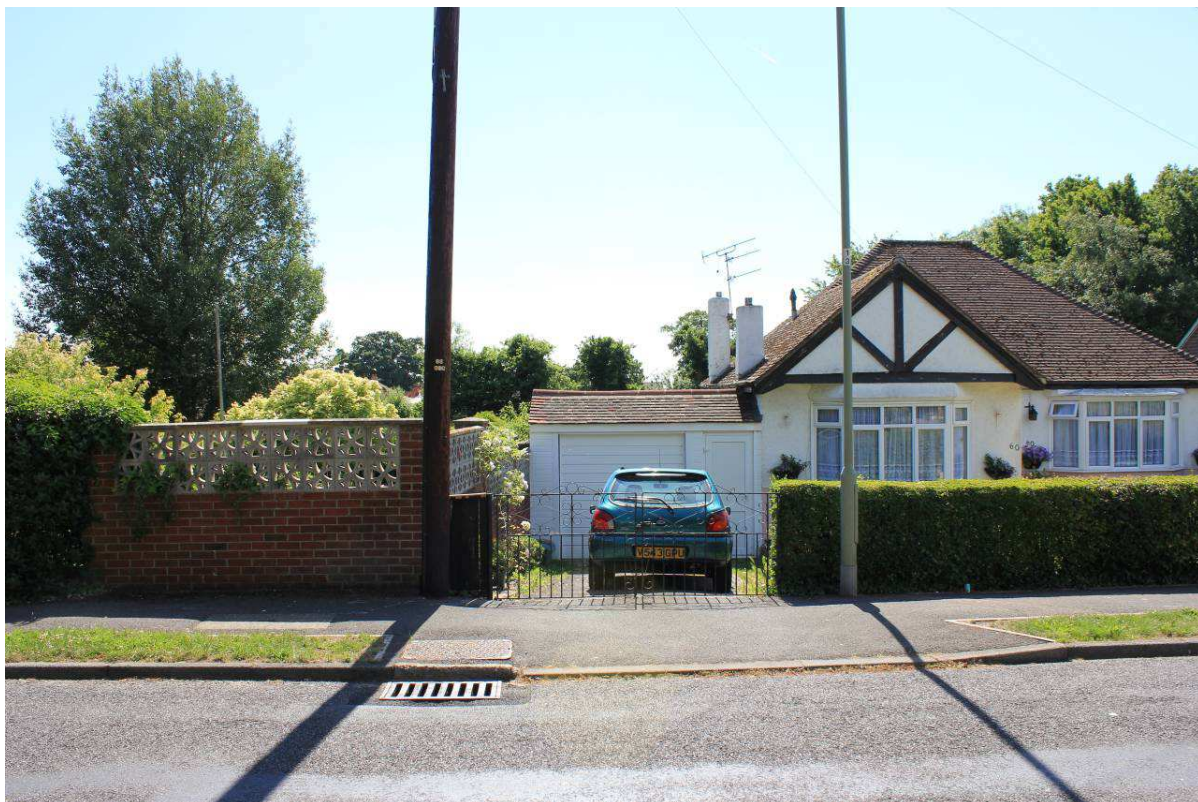
View of No. 60 Gladys Avenue from road (existing boundary hedge to plot on left).
