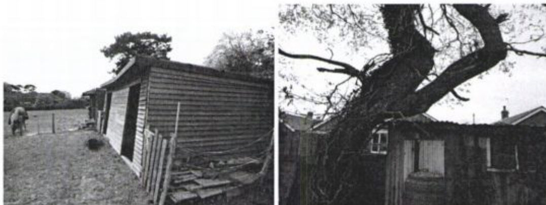
Buildings generally unsuitable for roosting bats
