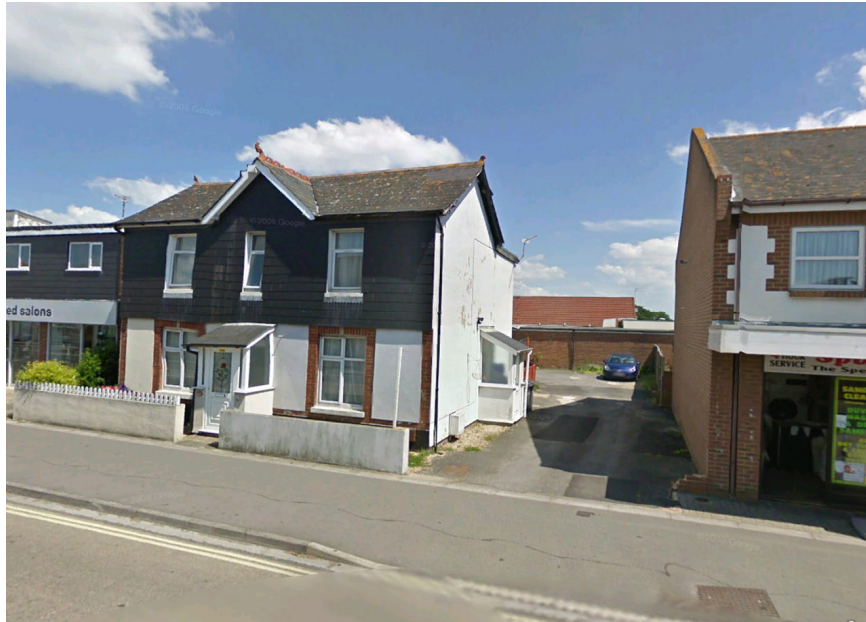
Fig 2 View from Elm Grove looking east
