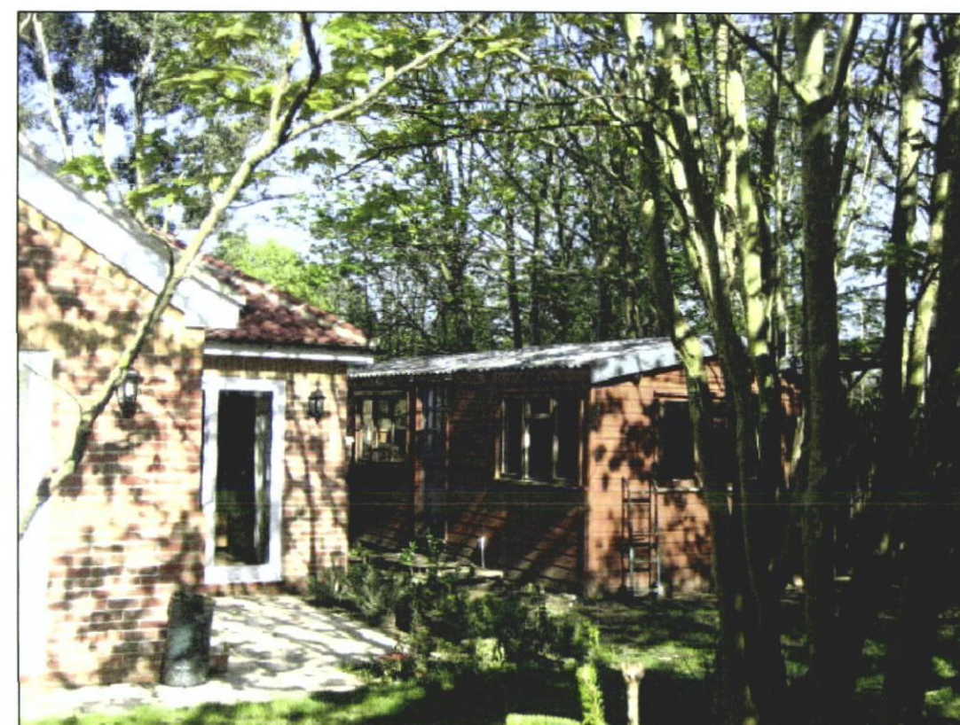
01 - View from SW from within Site
