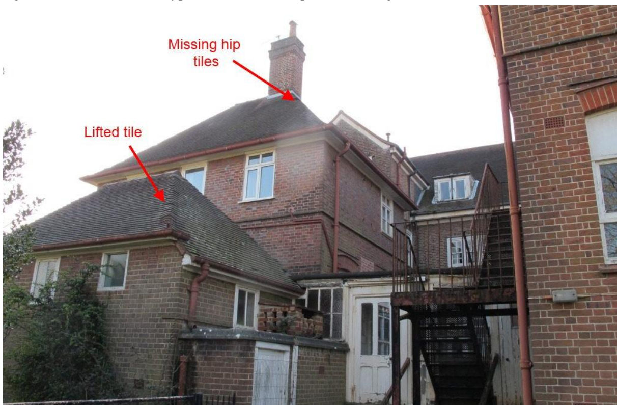
Figure C.7.1.13. Location of potential bat access points Building G.
