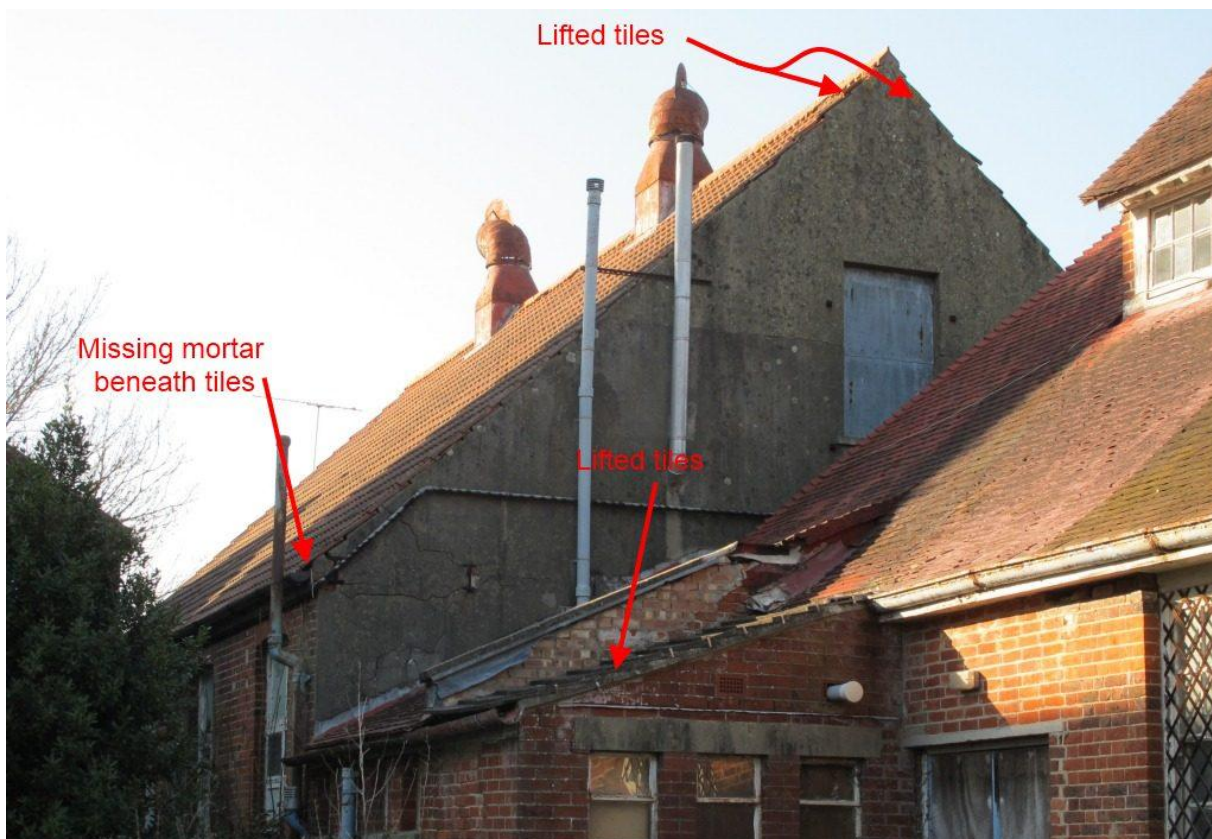
Figure C.7.1.7. Location of potential bat access points on Building B.
