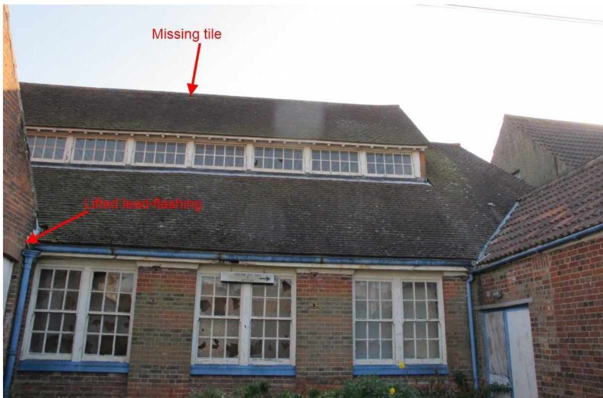
Figure C.7.1.5. Location of potential bat access points on Building B.
