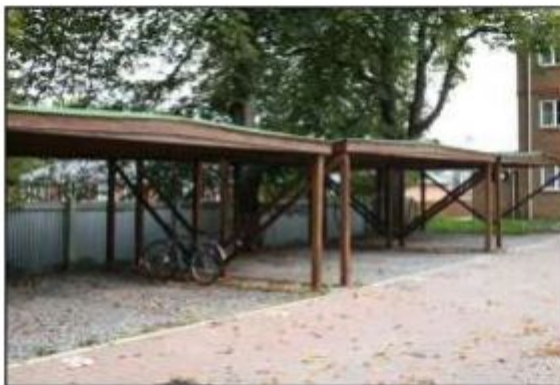
Photo 34: These carports are formed by wooden posts above a three dimensional cellular no-dig and load-spreading surface of permeable crushed stone.
