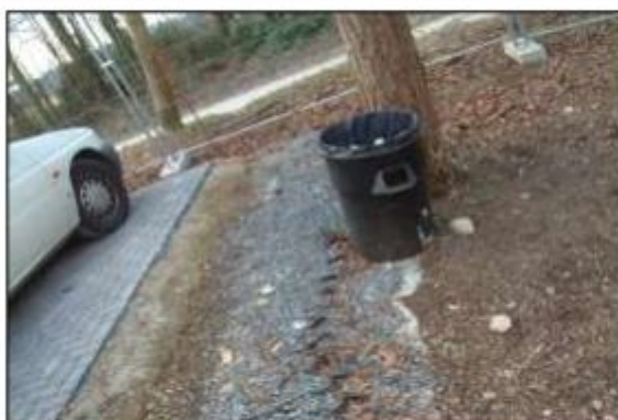
Photo 26: A conventional concrete haunching can be used to retain new surfacing as long as it is not dug into a trench - here it is placed on top of the CelWeb layer.
