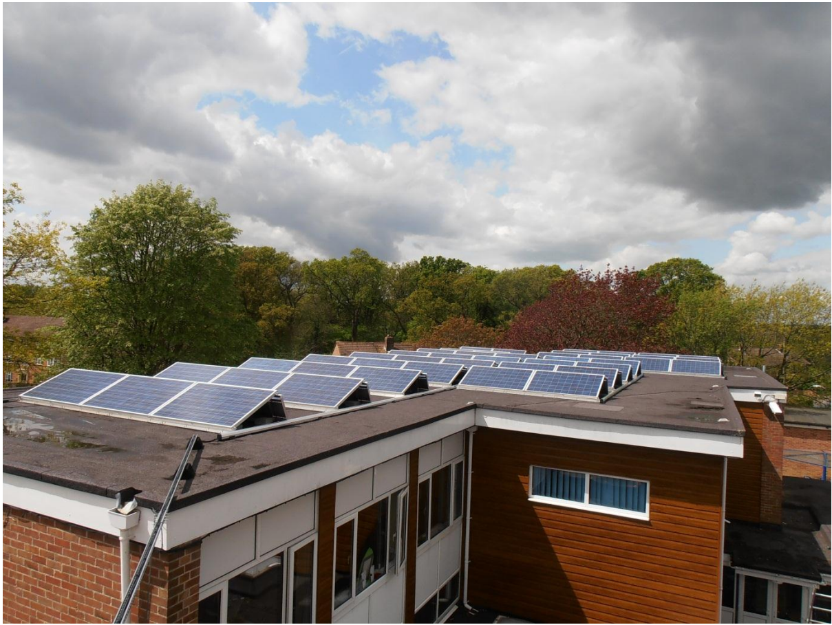
Image 2: Finished installation on the roof of Front Lawn Junior School
