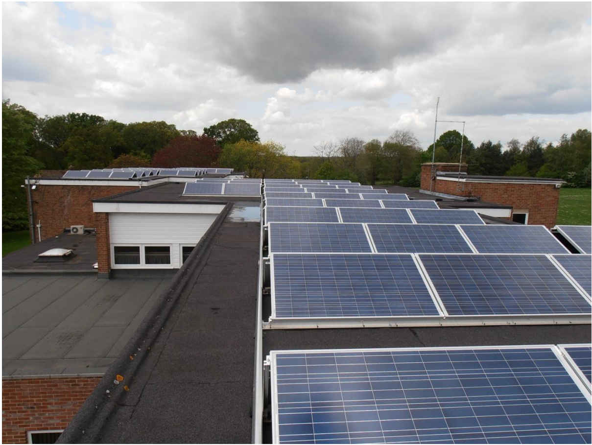
Image 3: Finished installation on the roof of Front Lawn Junior School
