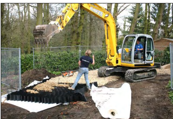
Photo 11: Cellular products are a very effective means of providing ground protection where heavy vehicle use is expected. Here, it is being used to temporarily widen an existing road, to be removed once the construction is finished.
