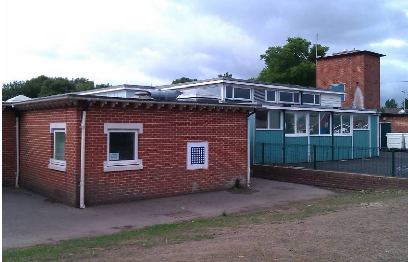
Plate 3 – School buildings on site
