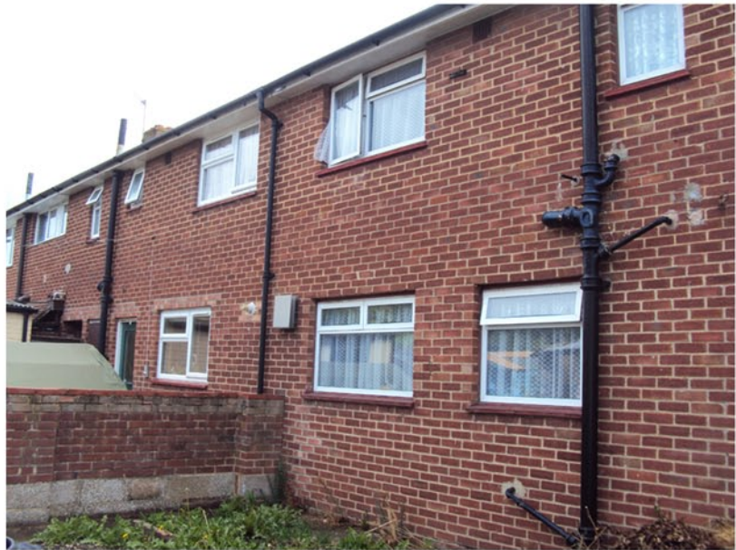
Rear of house (west elevation)
