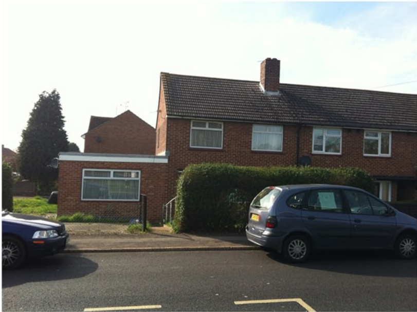
Front of house and view from St. Albans Road
