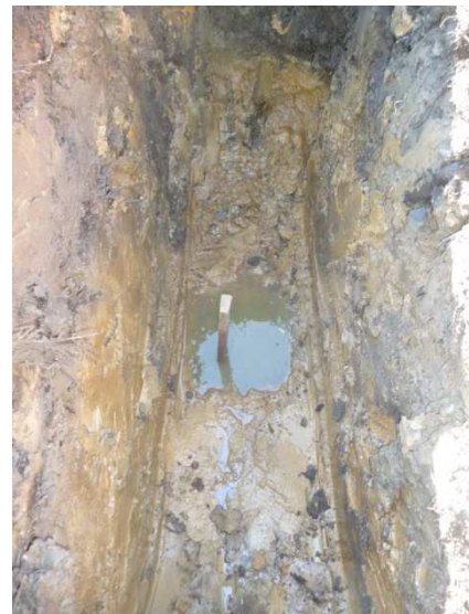
Excavation A end of percolation test
