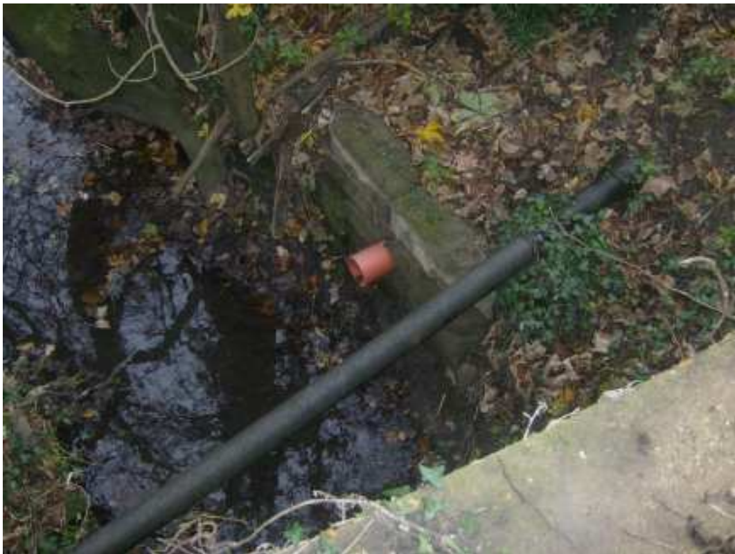
EXISTING STORM OUTFALL TO HERMITAGE STREAM
