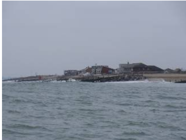
Receptor 7 – Viewpoint 19 Looking west at existing rock/timber groynes
