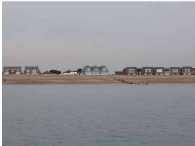
Receptor 7 – Viewpoint 21 Looking North – Bosmere road accessway is to the right of the distinctive blue 3 ridged roof house.
