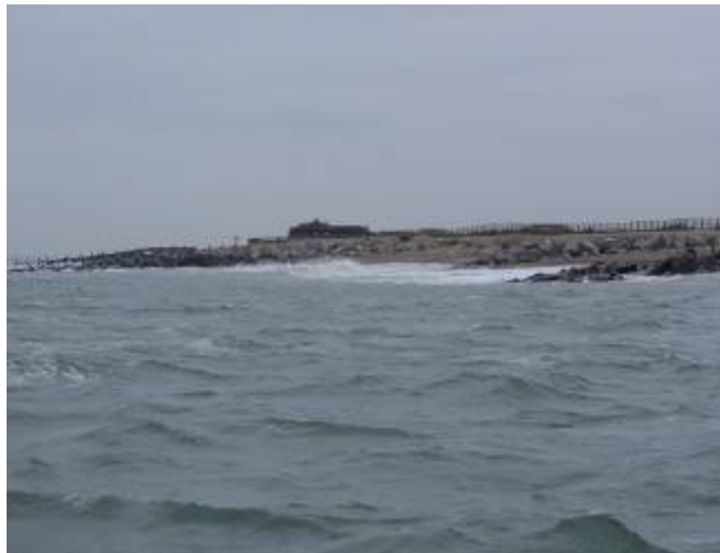
Receptor 7 – Viewpoint 20 Looking west at existing rock groynes
