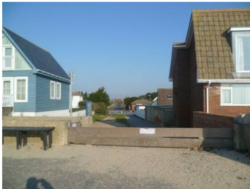
Image1 Storm boards point at Bosmere Road
