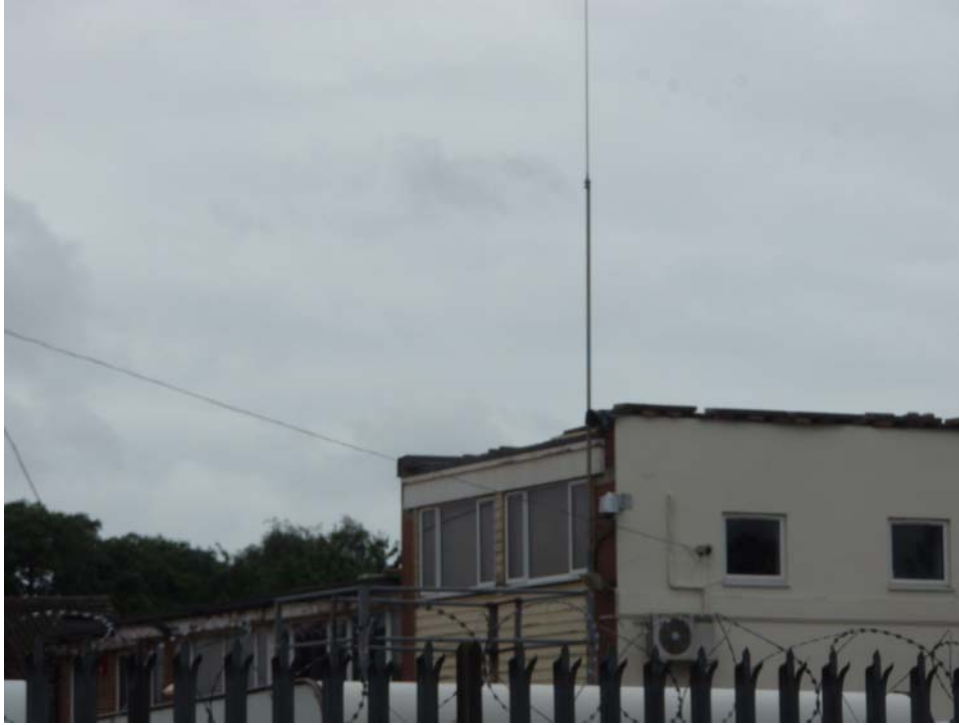
Photograph 4 – 'Havant Cabs' radio aerial.
