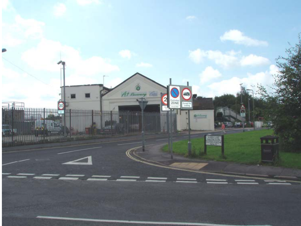
Photograph 5 - Elevation of the site from Eastern Road.
