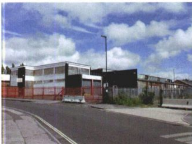
Site 23: 1 Silverthorne Way, Waterloooville
