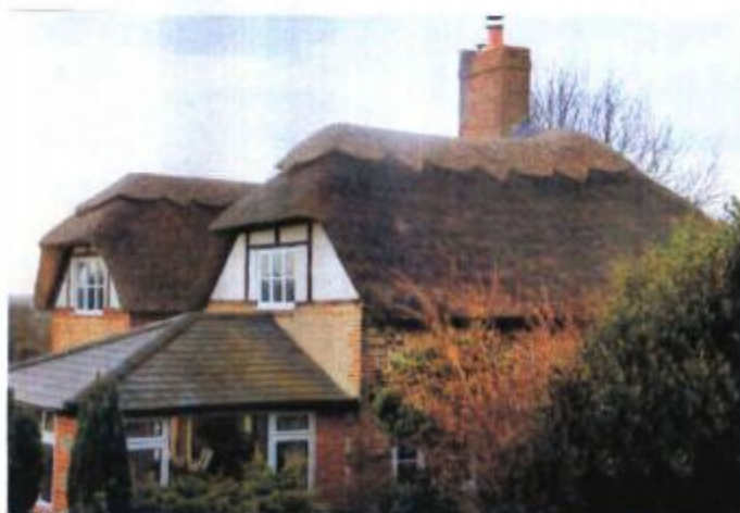
Fig 5: Two different roofs: Combed Wheat on left, Water Reed on right
