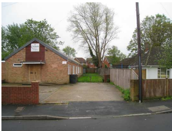
The application site viewed from Kings Road (north)
