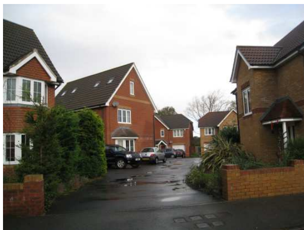
The application site viewed from Pepper Close (south)
