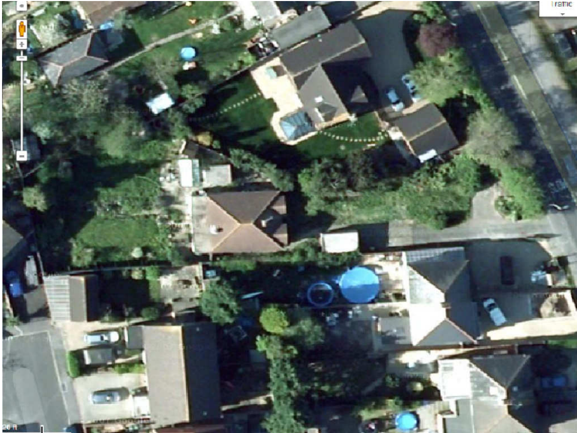
Aerial View of 41 Hulbert Road (Google Earth Image)
