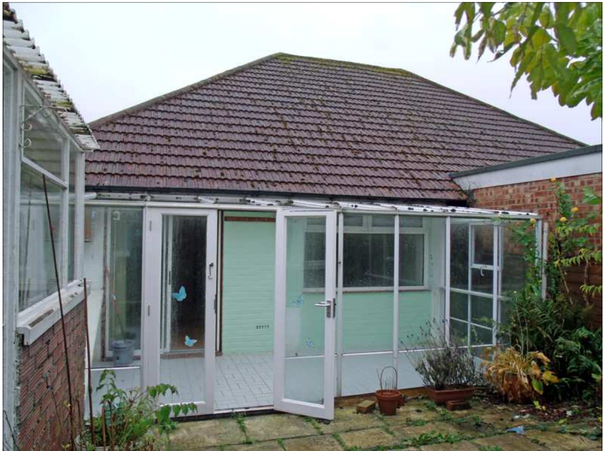
Rear of No. 14 showing conservatory and corner of greenhouse
