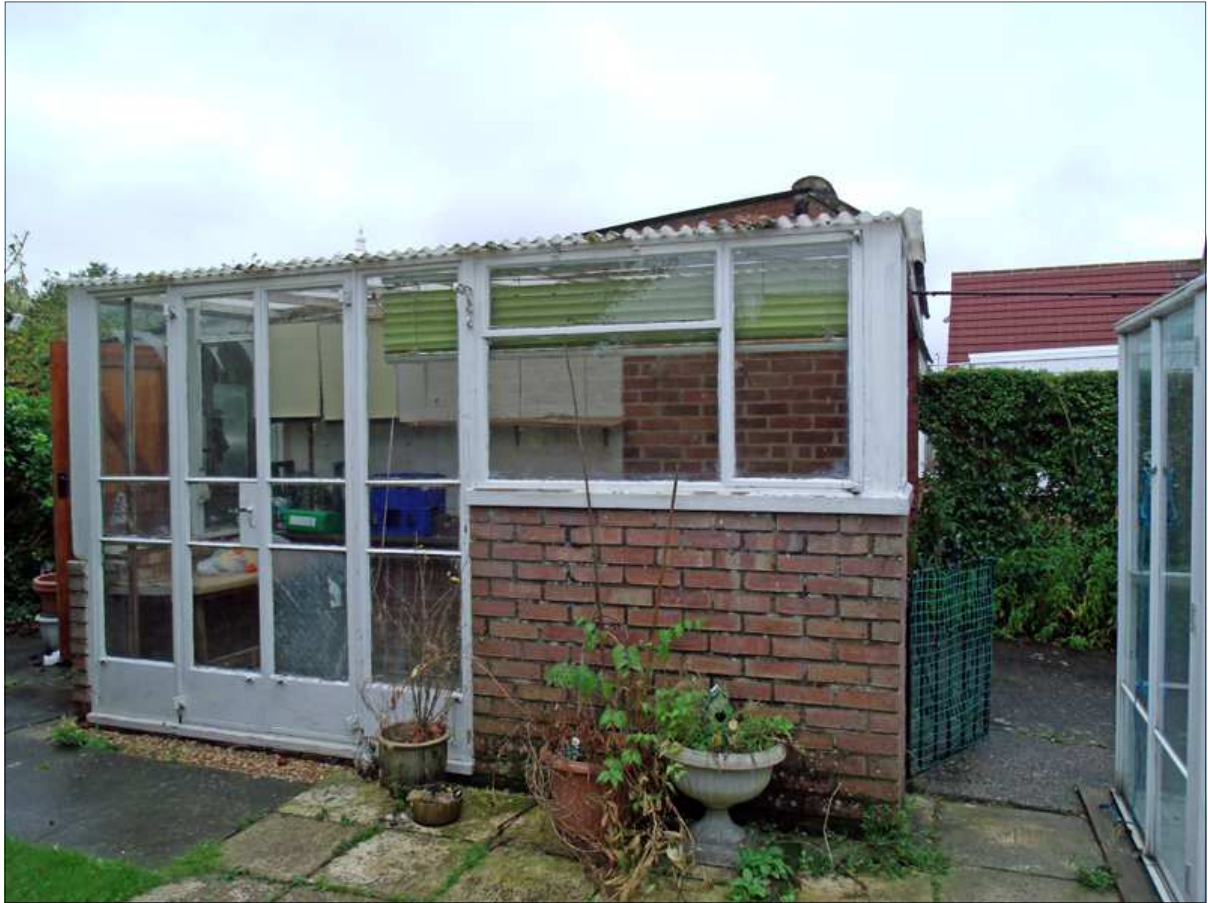
Former greenhouse at No. 14
