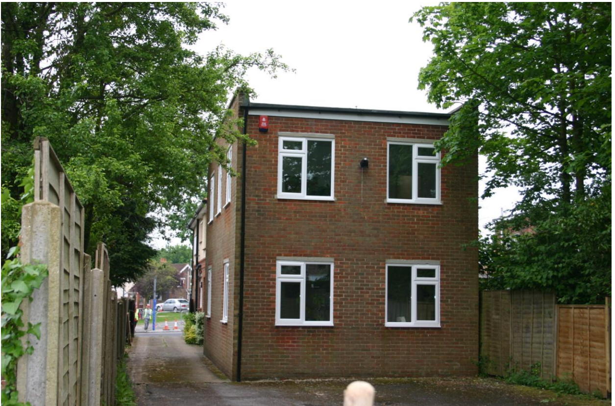
Office building to south, fronting London Road.
