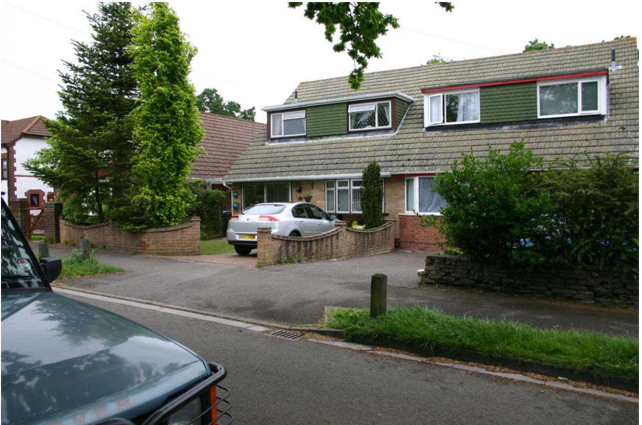
View of 2 & 4 Summerhill Road with no on-site turning.
