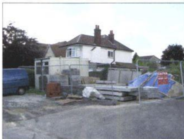
Construction site of replacement house (no. 48) to North of the site (pictured 12.10.2012)
